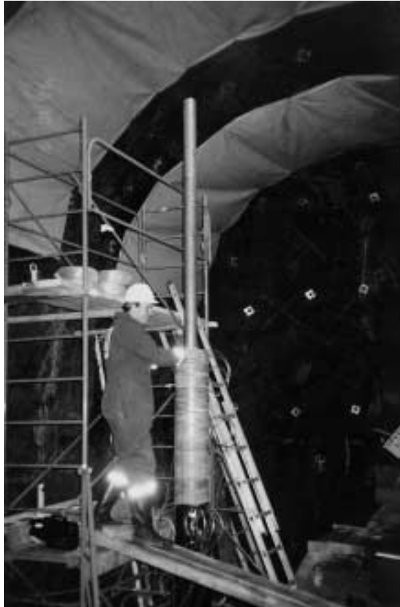
Figure 4-1 Mounting of the S1 parcel at test site.
