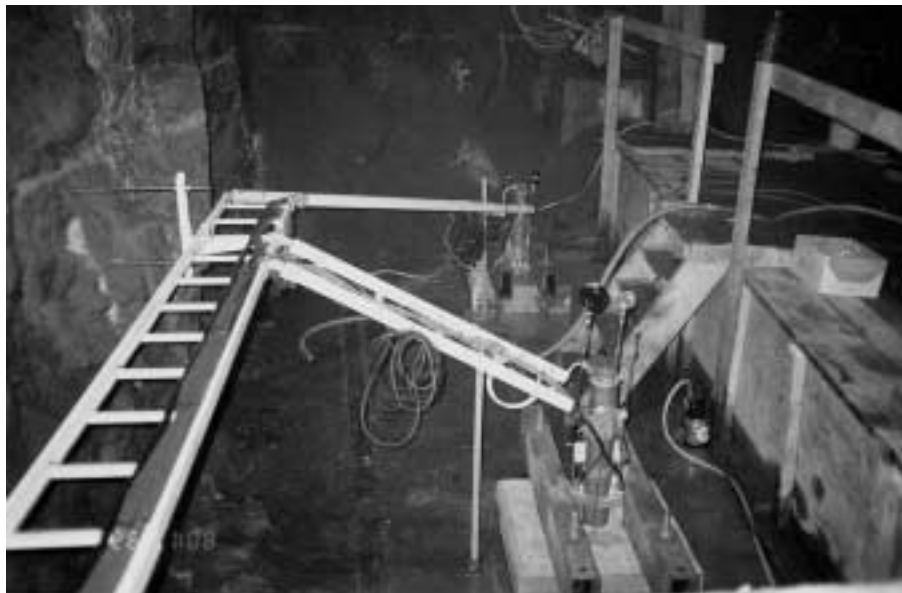
Figure 4-2 Final appearance of the pilot test site after installation.
