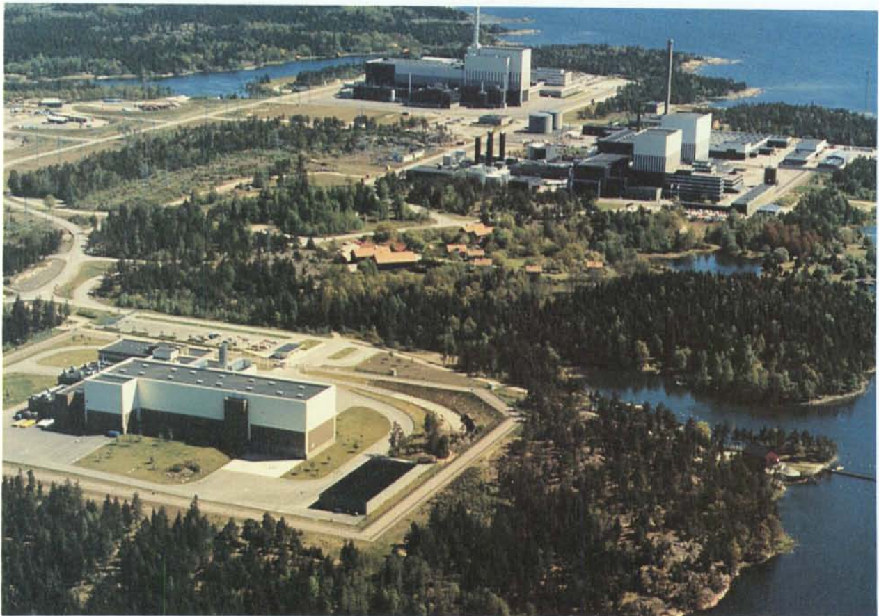
Figure 3-1. The Oskarshamn Nuclear Site. CLAB in the foreground.
