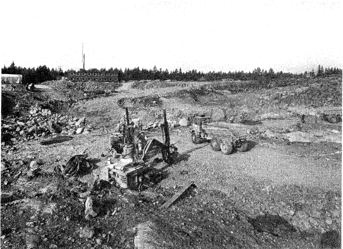
Figure 3. Worksite for Clab, 29 September 1980
