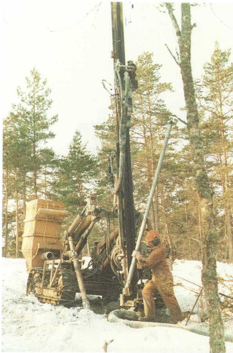
Figure 4.2 Percussion drill rig.
