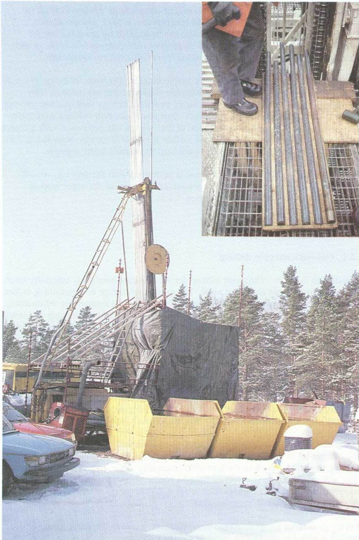
Figure 4.3 Core-drilling rig and pieces of core.
