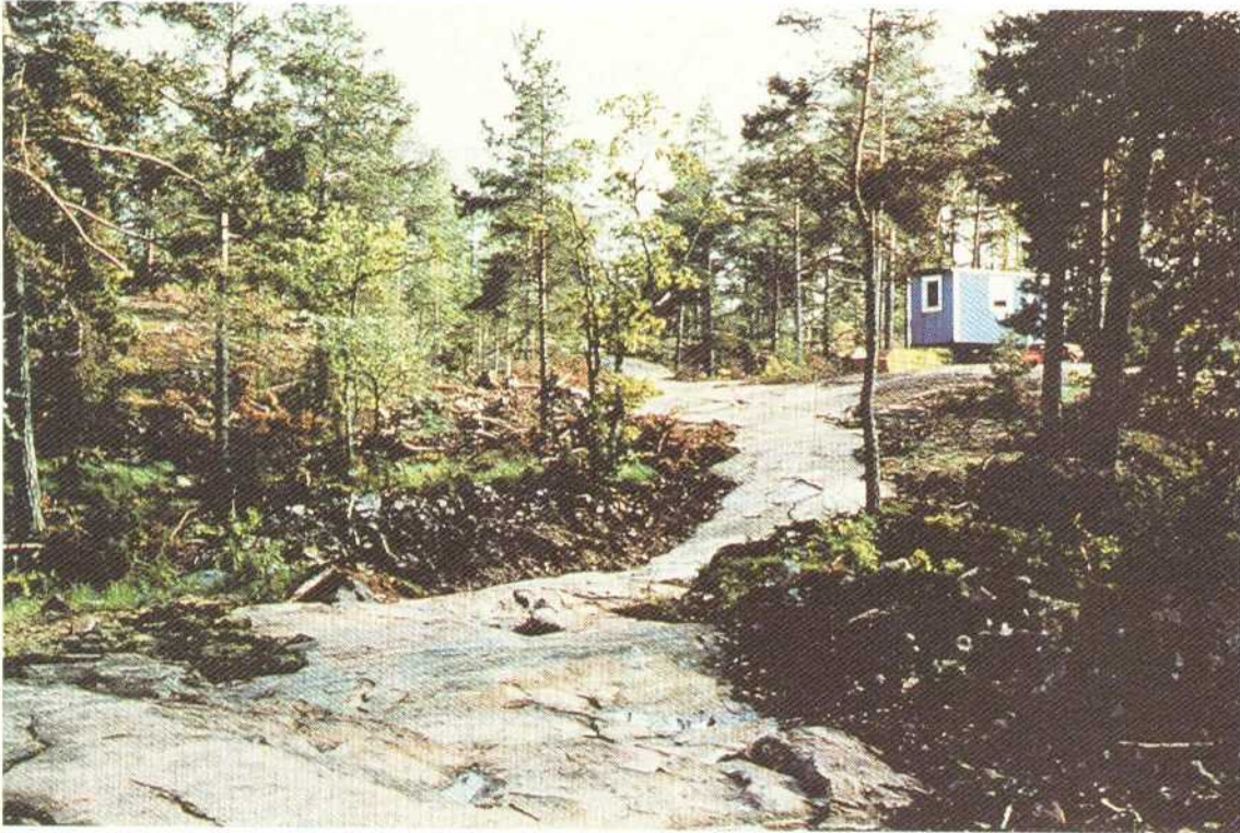
Figure 3.3 Trench on the Äspö island, where the thin layer of overburden was removed for detailed geological mapping.
