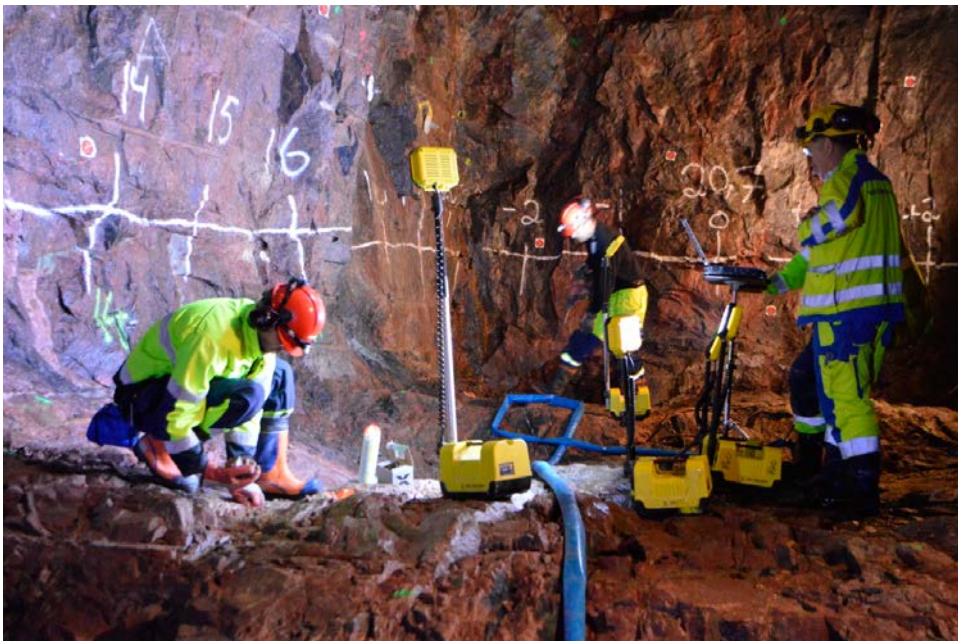
Figure 4-29. Mapping of TAS06 and identification of suitable positions for the deposition holes.
