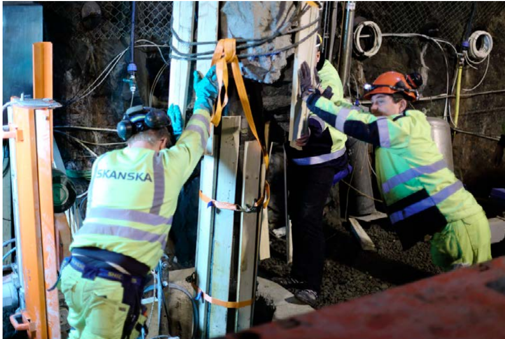
Figure 4-7. Excavation of the ABM2 experiment.
