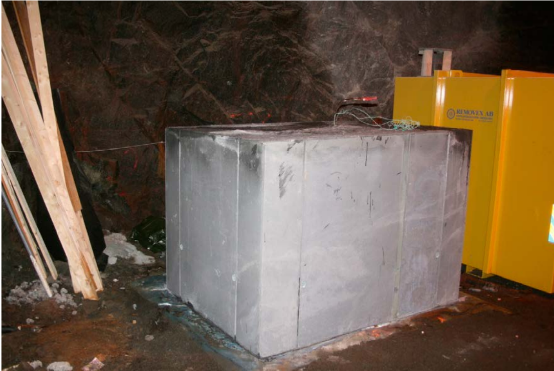
Figure 4-33. Monolite in low-pH concrete.
