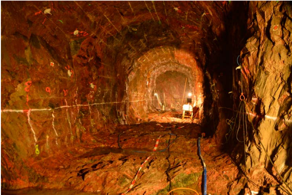
Figure 4-28. TAS06 after removal of rock debris and mud.
