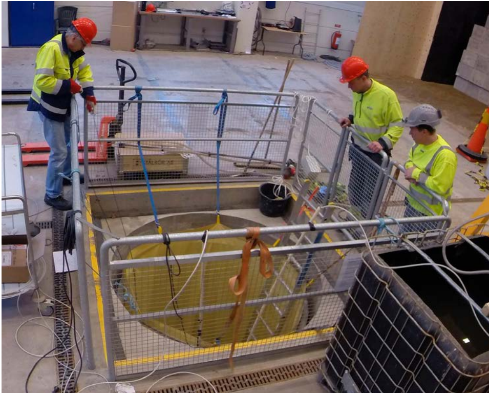
Figure 4-57. Photo taken when removing the o-ring.
