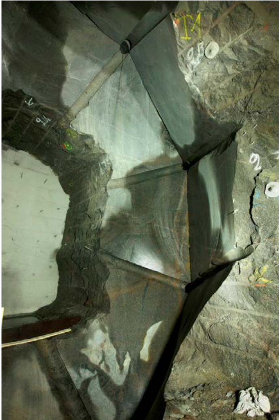
Figure 4-44. Part of the concrete dome abutment, excavated by wire-sawing.
