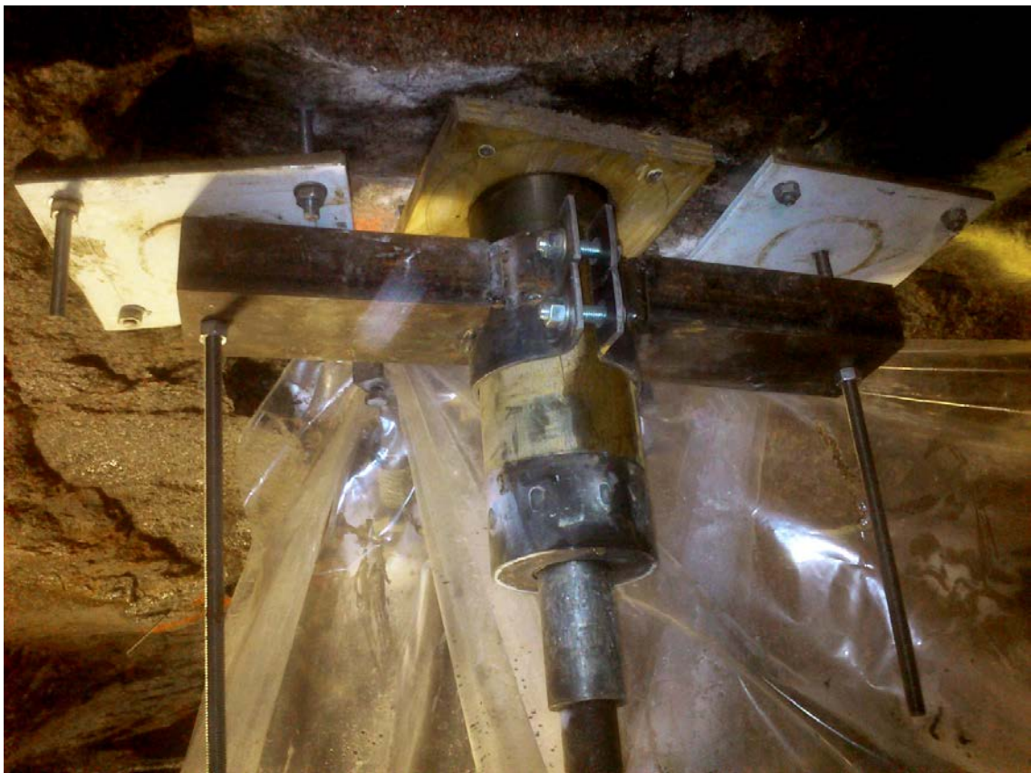
Figure 4-35. Overcoring of a vertically emplaced rock bolt.
