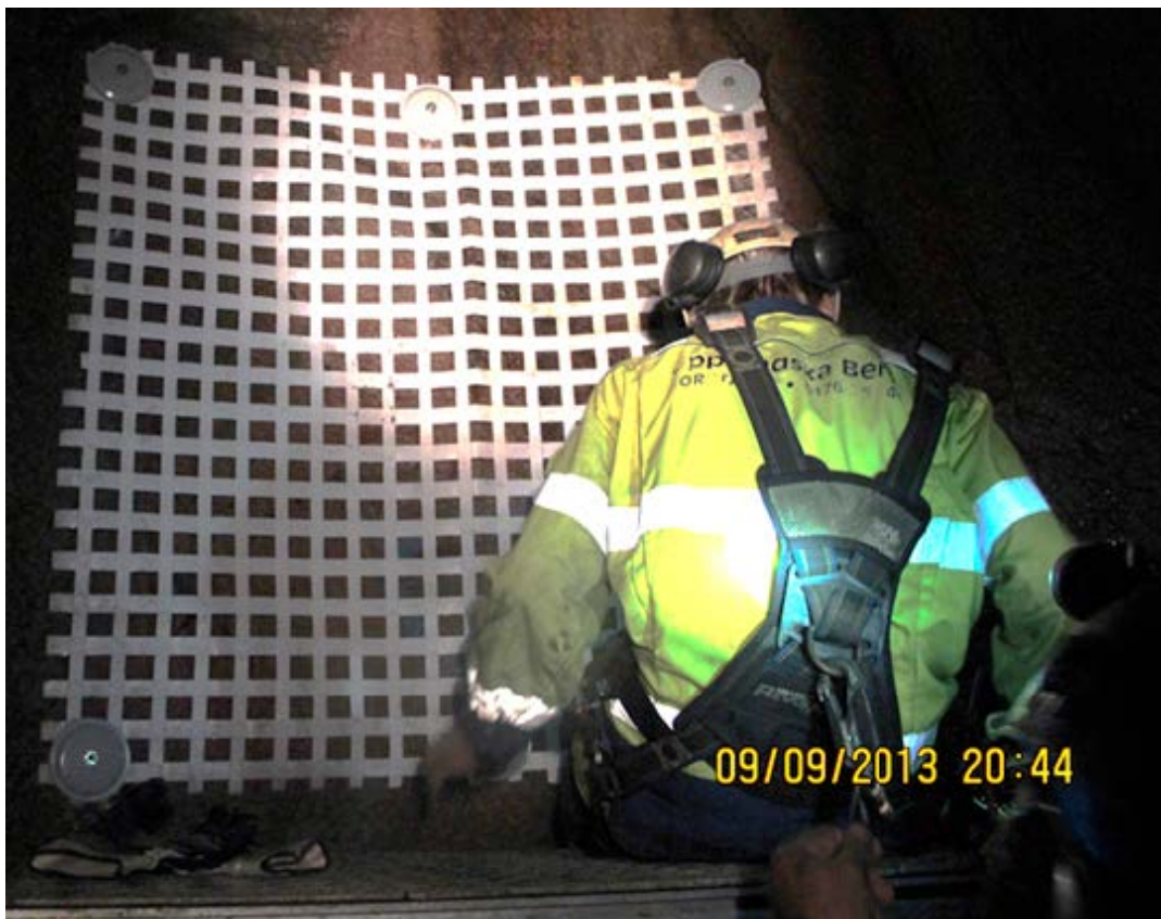
Figure 6-4. Reinforcement of the elevator shaft using netting and expansion bolts.
