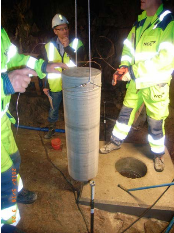
Figure 4-26. Installation of the first concrete cylinder in NASA 2861A.
