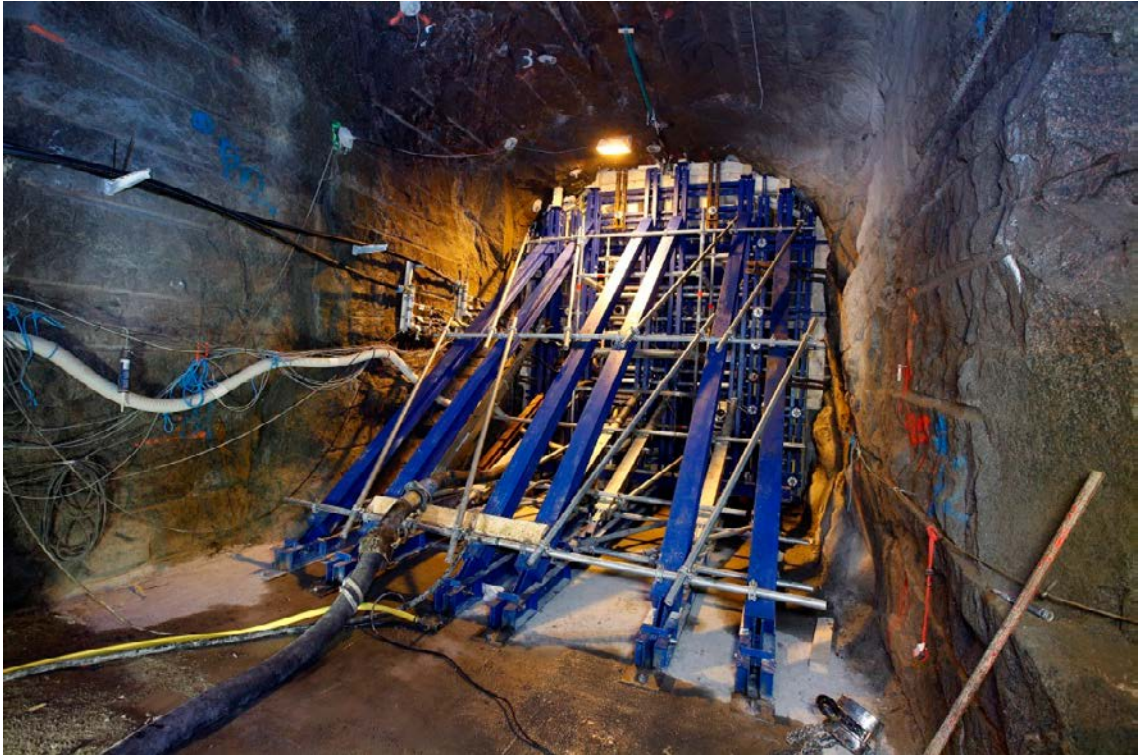
Figure 4-47. Formwork for casting of the concrete dome structure.
