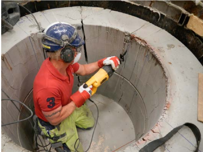
Figure 4-53. Dismantling of the test.
