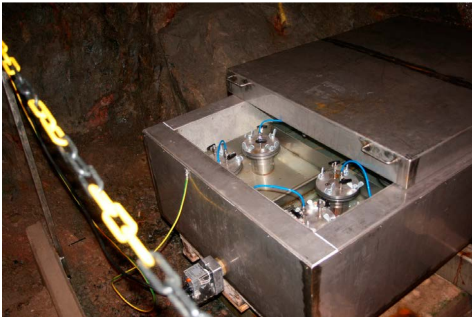
Figure 4-27. The steel cylinders stored at about 50°C in water in NASA2861A.
