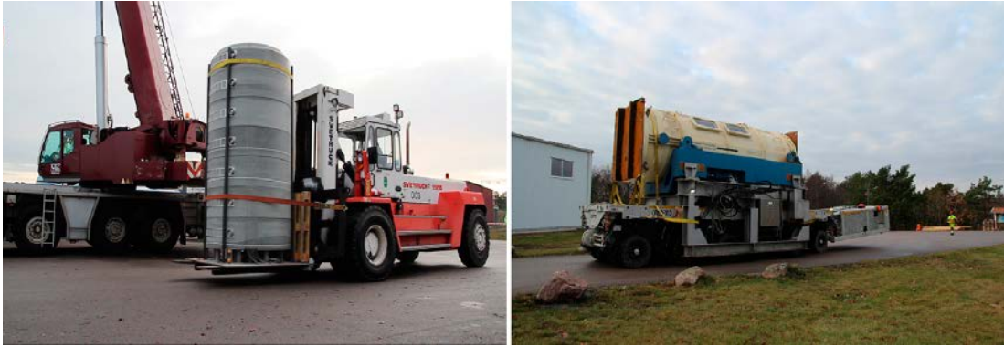
Figure 4-15. To the left, the assembled distance block is moved out of the assembly hall. To the right it has been placed in the transport tube and is moved using the heavy load vehicle MODE.
