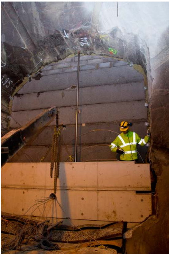
Figure 4-46. Installation of concrete delimiters, bentonite seal, macadam filter and sensors.
