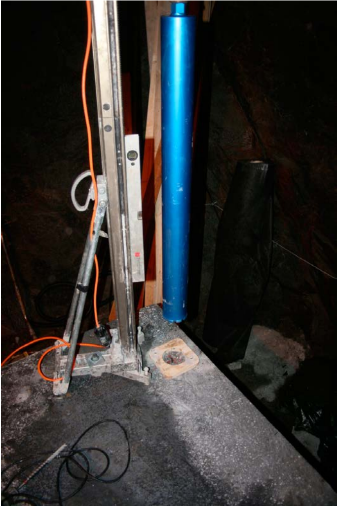
Figure 4-37. Concrete cores are taking out of the monolite.
