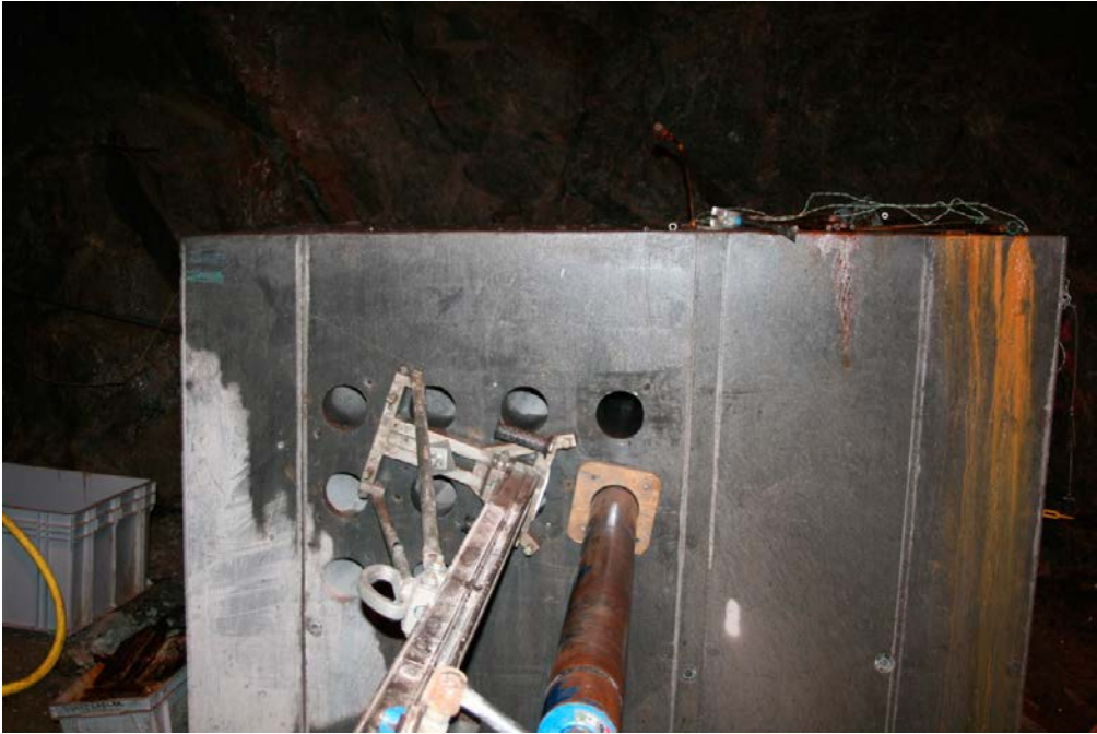
Figure 4-36. Concrete cores are taking out from the monolite.
