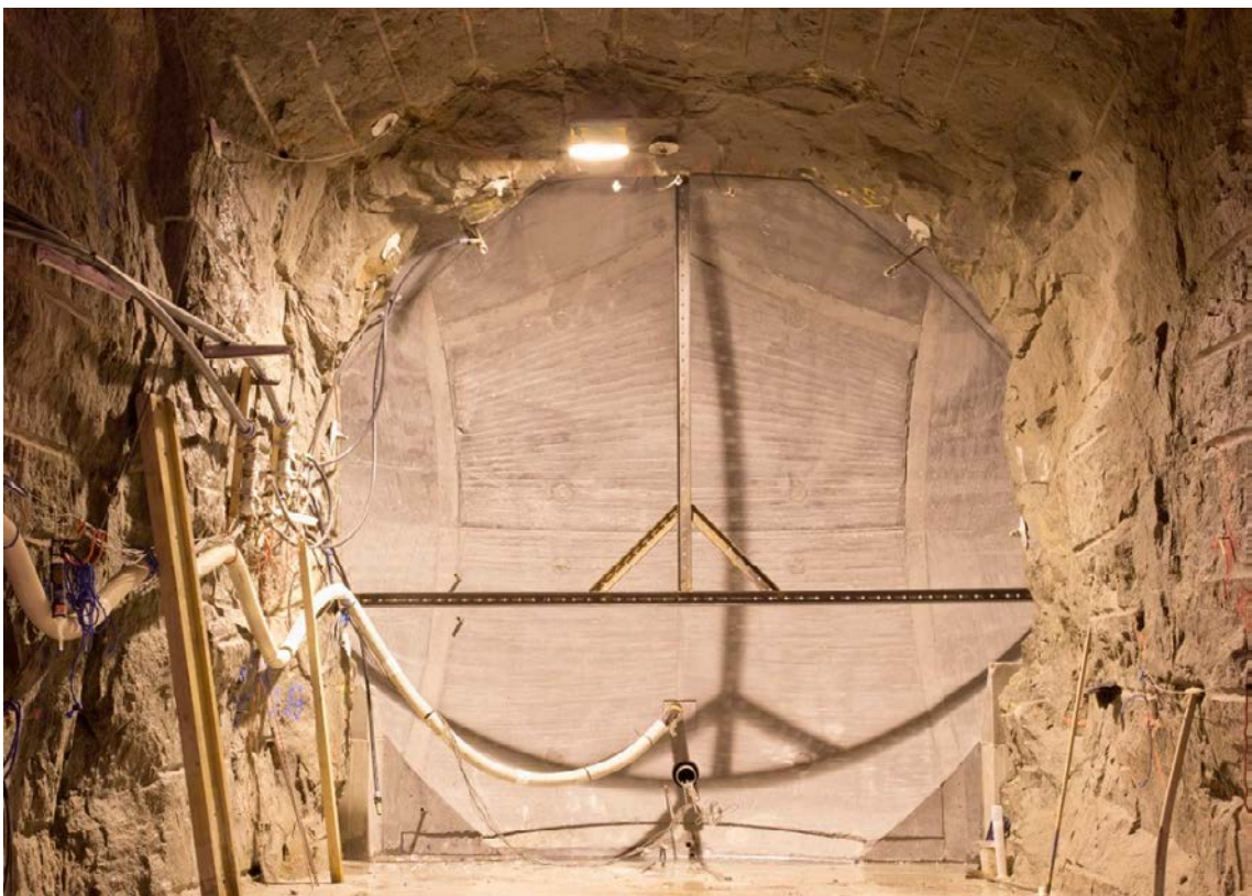
Figure 4-48. The concrete dome structure after removed formwork.
