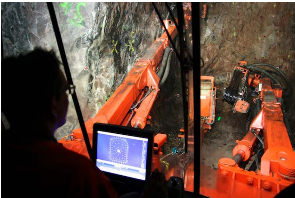
b) View from the operator's cab of the Sandvik drill jumbo. The computer screen with the blast hole layout can also be observed.
