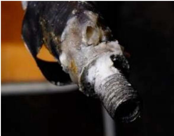
Figure 6-14. Galvanic corrosion between Aluminium (rod) and stainless steel (junction).
