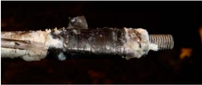
Figure 6-19. Severe corrosion under the PVC-tape in the inner anaerobic zones (KA3385A and KA3105A). This photo is from KA3385A, area 1, section 1.
