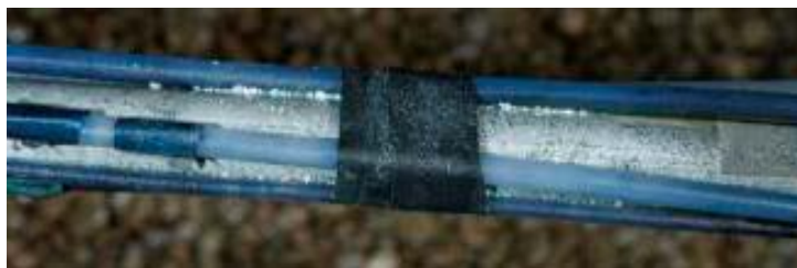
Figure 6-23. Corrosion under tubing.
