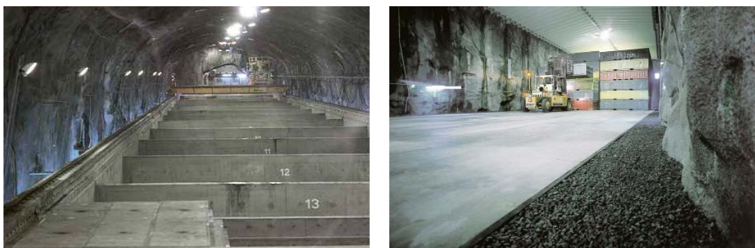
Figure 2-2. The rock cavern for intermediate level waste, BMA, in SFR (left) and the rock cavern for low-level waste, BLA, in SFR (right).
