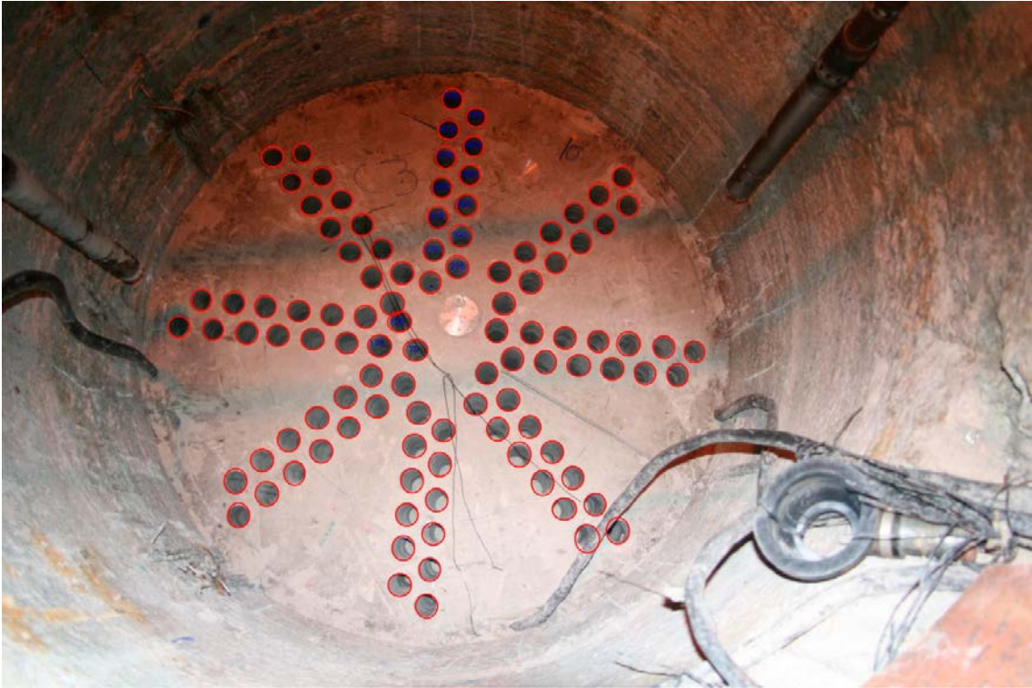
Figure A2-9. Block No C3 deposition hole 5.
