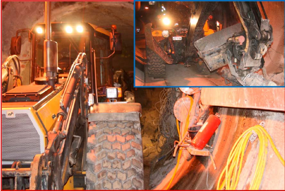
Figure 3-2. The backhoe loader used at the excavation.
