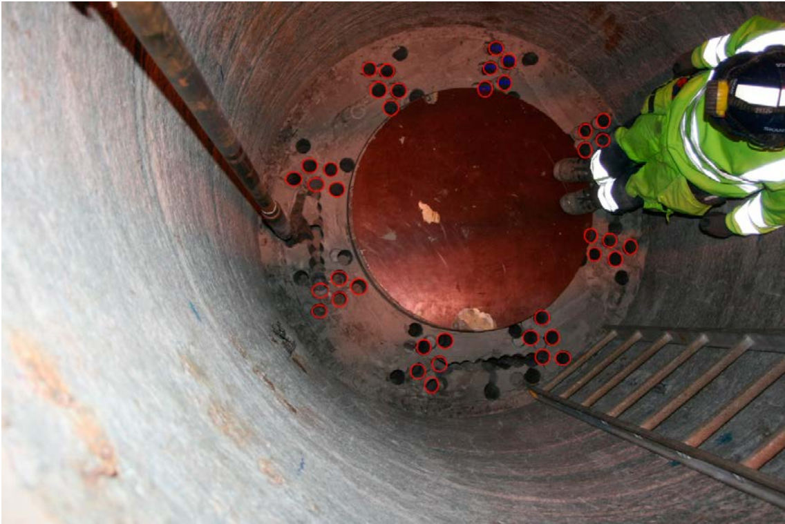
Figure A2-6. Block No R9 deposition hole 5.
