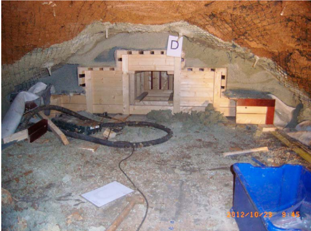
Figure 5-4. Photo taken during the excavation of the bentonite pellets.
