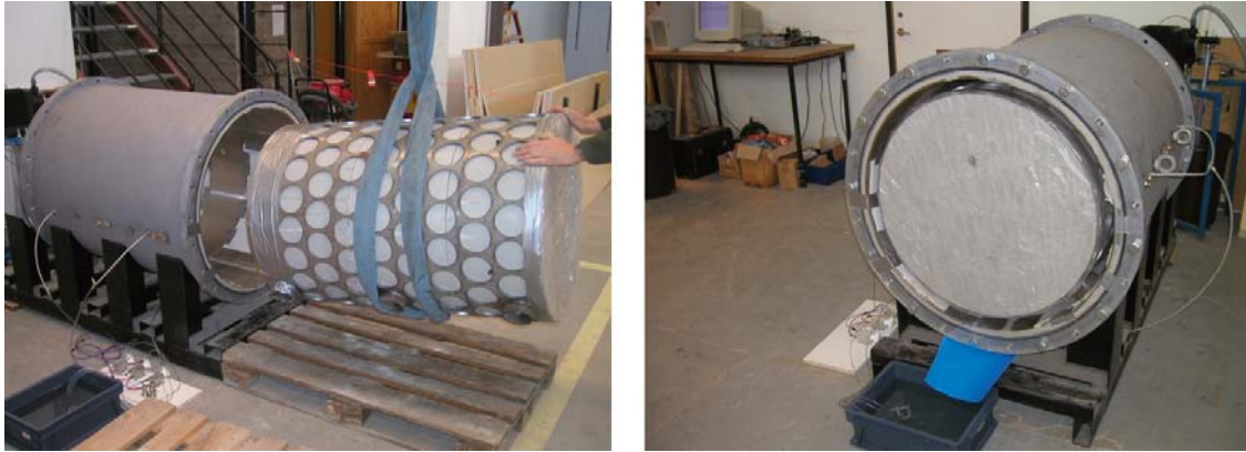
Figure 5-9. Installation of Supercontainer simulator. (Left: The open end of the Supercontainer was covered with plastic to minimize atmospheric interactions. Right: Plexiglas lids mounted in the ends to allow visual monitoring of bentonite block behaviour.
