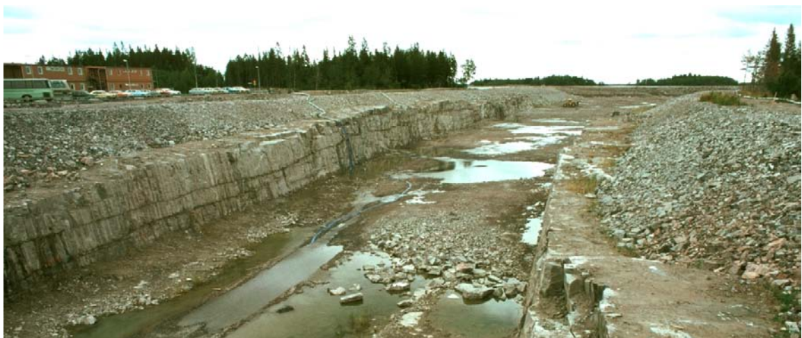
Figure 3-7. The canal between the nuclear power reactors and the Baltic Sea exposing extensive undulating sheet joints. Taken from Carlsson och Christiansson (2007). Photograph by G Hansson.
