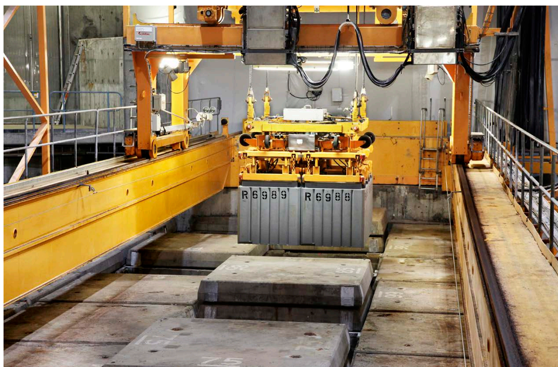
Figure 2-8. Disposal of waste packages (steel moulds) in the silo.
