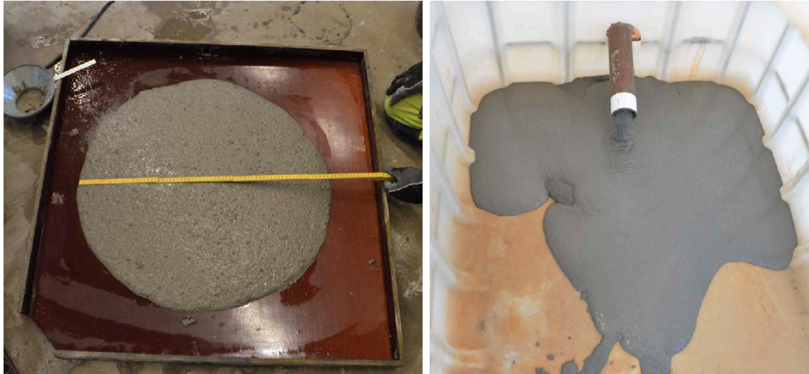
Figure 3-5. Measurement of the flowability of the SFR borehole concrete (left image) and testing of concrete pouring using the drill tube (right image).
