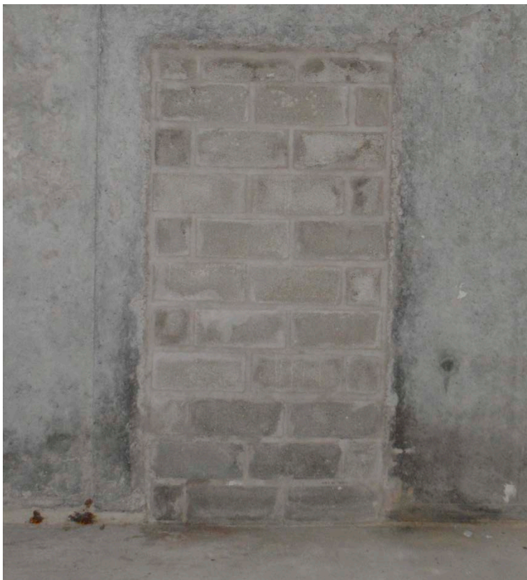
Figure 2-13. Sealed doorway in the inner wall separating two adjacent waste compartments.
