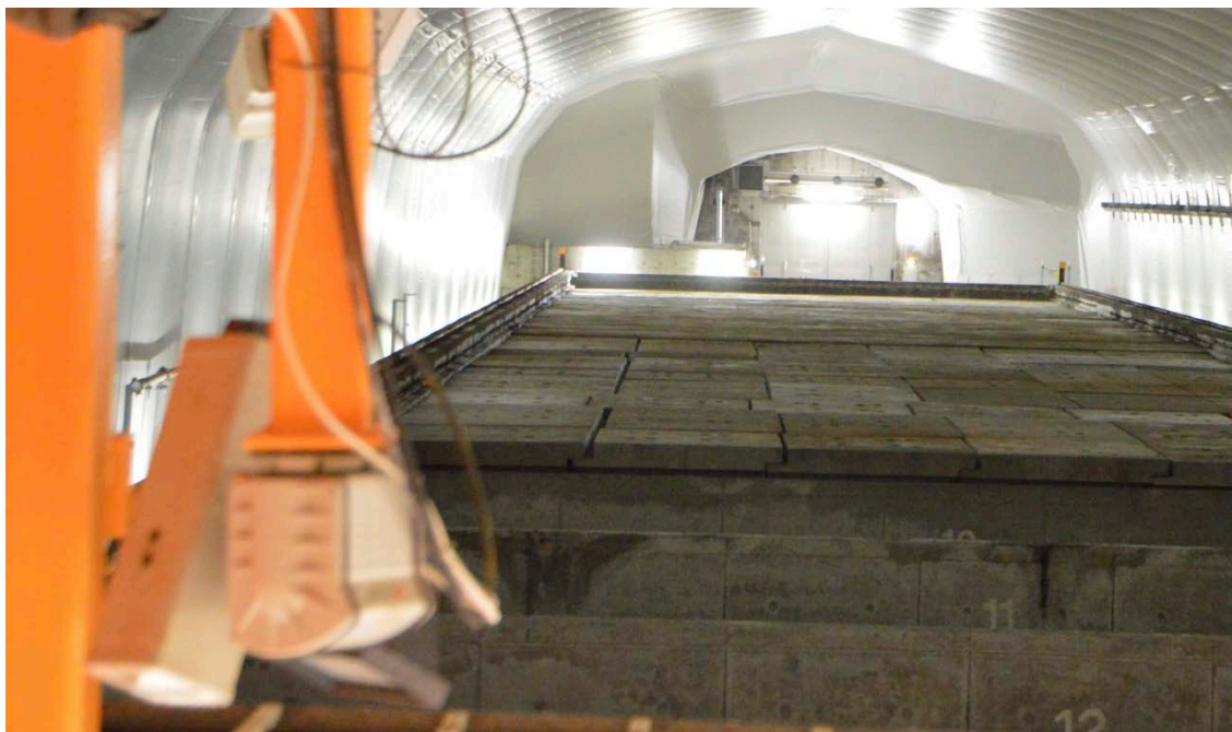
Figure 2-14. Waste vault for intermediate-level waste, 1BMA, during the operational period. Note the different states of the different compartments. Those in the farthest part have been entirely filled with waste and provided with concrete elements for radiation shielding and a thin layer of concrete. The compartments in the middle have been filled with waste and covered with radiation shielding concrete elements while no waste has yet been disposed in the nearest compartments.
