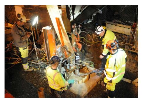
*Figure 4-11.* Photo showing the released test package. After the seam-drilling, two core drilled holes with a diameter of 300 mm were drilled in order to make it possible to install the wire-sawing equipment and saw off the rock column at the bottom.
