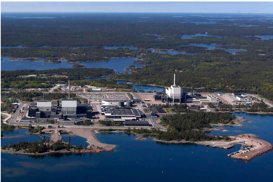
Figure 15-3. View of OKG Aktiebolag's nuclear power plant with the three BWR reactors O1, O2 and O3 from left to right in the picture.
