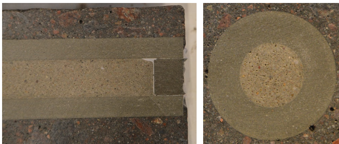
Figure 9-2. Cross-section of a drill core from testing of different concepts for facilitating the use of tie rods in the construction of formwork for external walls for the caissons in 2BMA (Mårtensson 2021a).
