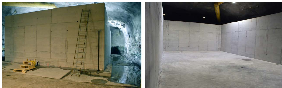
Figure 9-1. Cast caisson at the Äspö HRL, externally and internally (Mårtensson and Vogt 2020).
