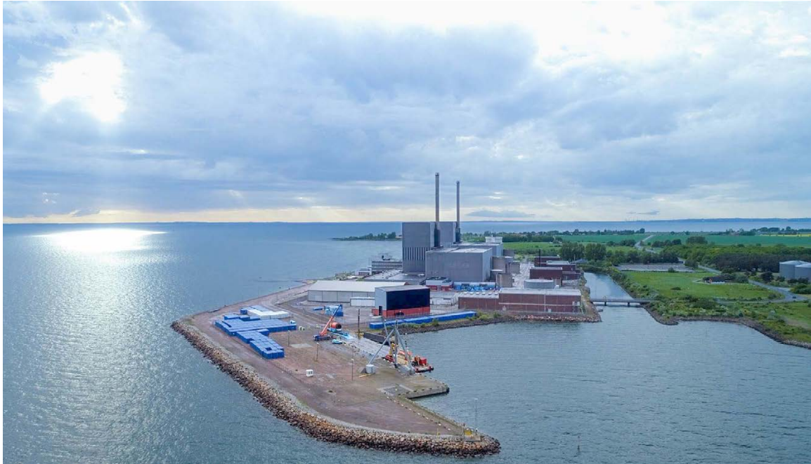
Figure 15-1. Barsebäck nuclear power plant viewed from the south with interim storage facilities in the foreground, Barsebäck 1 and Barsebäck 2 in the background. Photograph: Apelöga.
