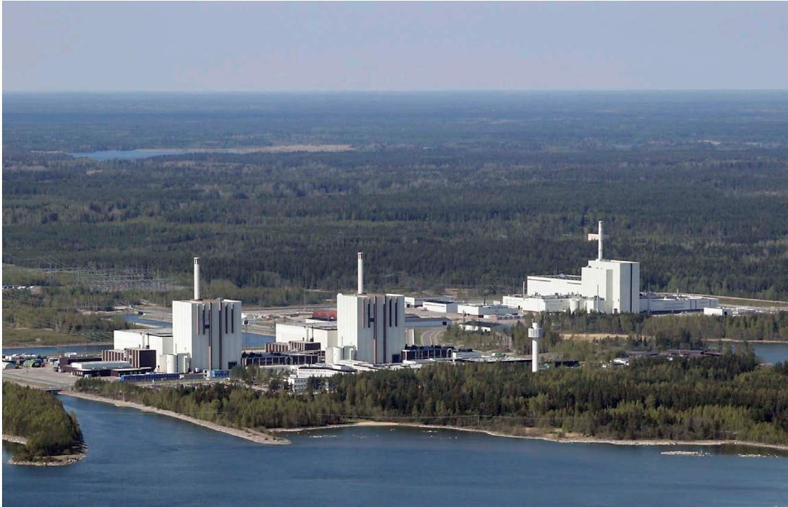
Figure 16-3. Forsmark power plant with the three BWR reactors F1, F2 and F3 from left to right in the picture.
