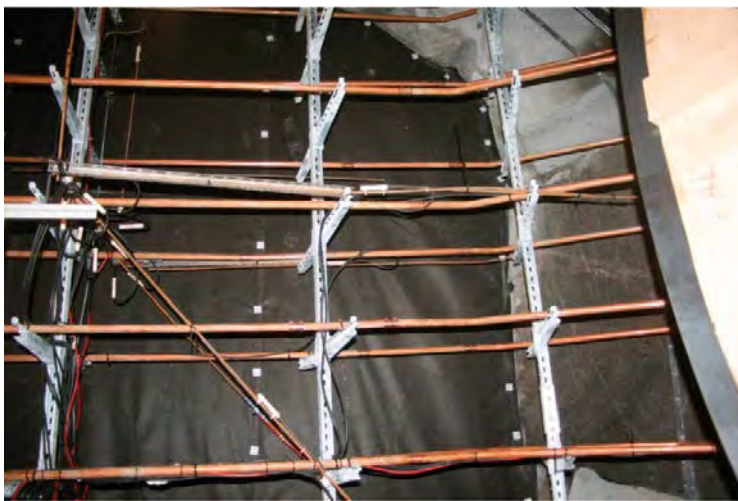
Figure 6-20. Installed cooling pipes with the supporting steel frame.
