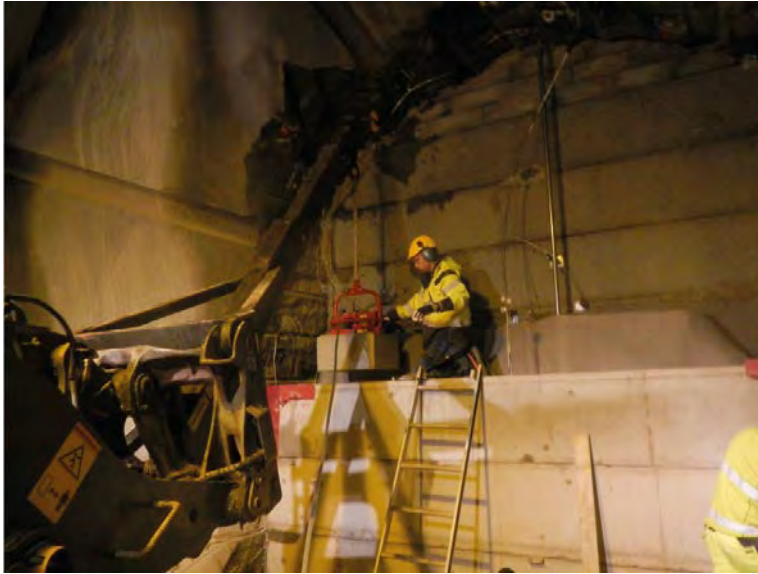
Figure 6-15. Installation of bentonite blocks for the DOMPLU bentonite seal.
