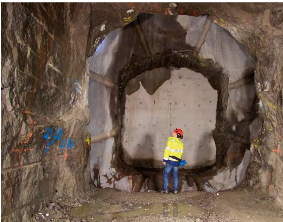
Figure 3-11. TAS01 with the excavated slot abutment for the concrete dome.
