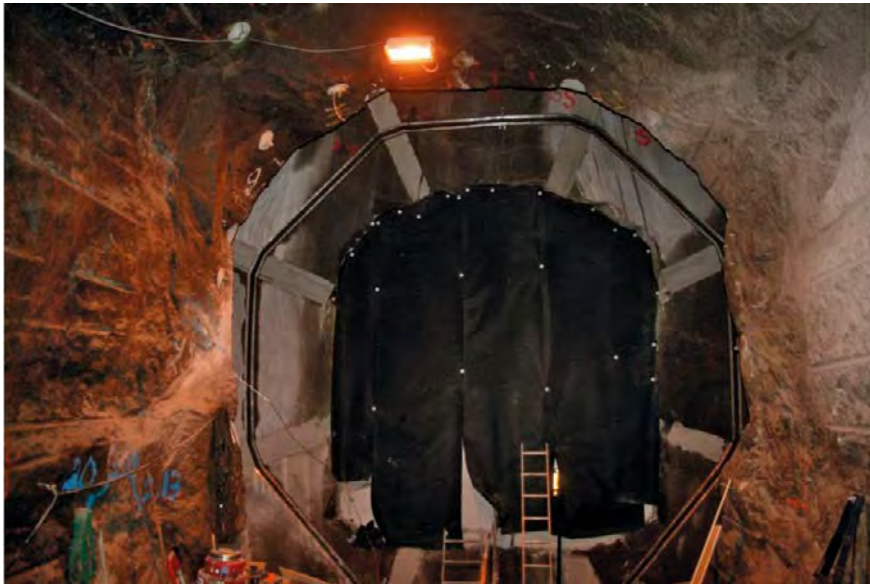
Figure 6-19. Geotextile fixed to the front of the concrete delimiter.
