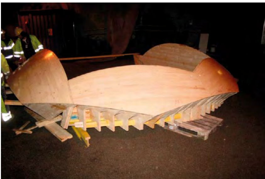
Figure 6-24. Prefabricated outer frame of the concrete dome formwork.
