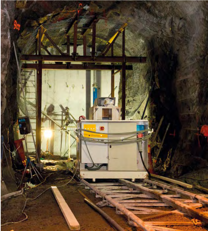
Figure 3-10. Wire-sawing equipment moving on rails in TAS01.
