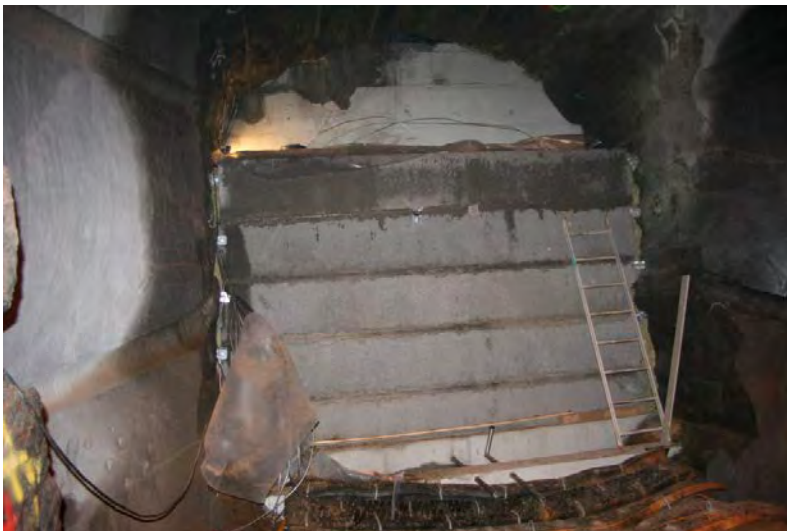
Figure 6-9. Installation of the LECA beams.
