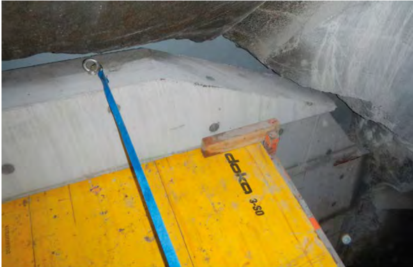
Figure 6-33. Photo showing the installation of the last concrete beam.
