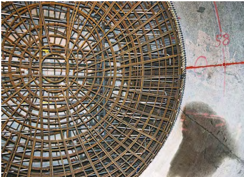
Figure 2-19. The outer reinforcement of the plug. (Figure 6-4 in Johannesson et al. 2004.)
