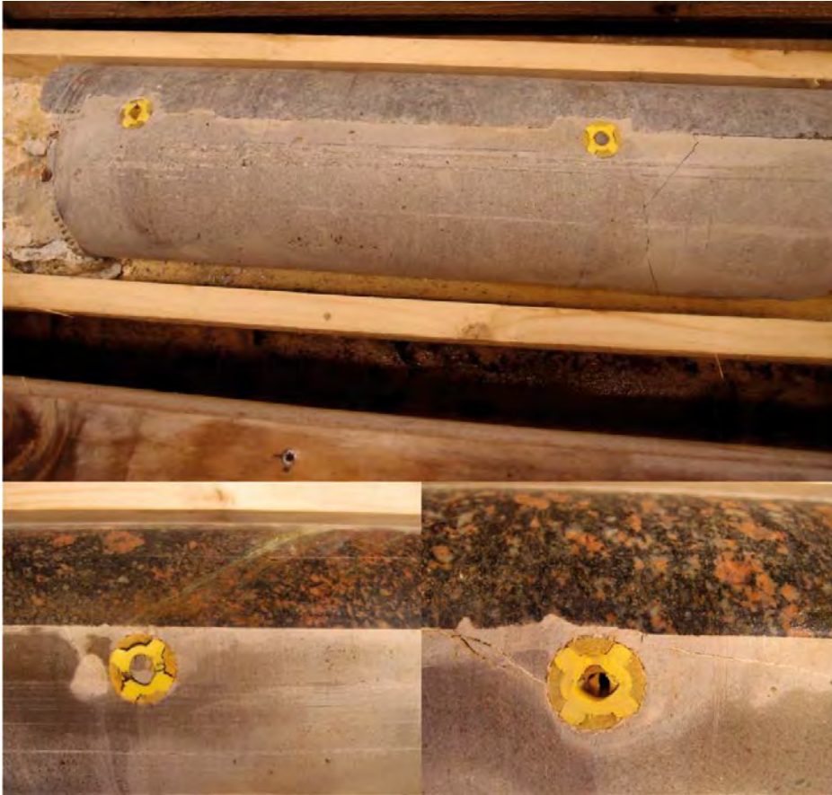
Figure 4-2. Close up pictures of the cores taken from the interface between concrete plug and rock. The yellow grouting tubes are embedded in grout. (Figure 2-6 in Johannesson and Hagman 2013.)
