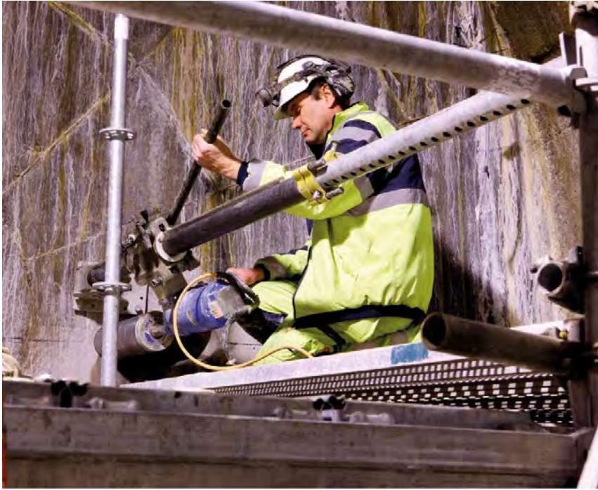
Figure 4-3. The rig used for core drilling through the concrete dome. (Figure 2-5 in Johannesson and Hagman 2013.)
