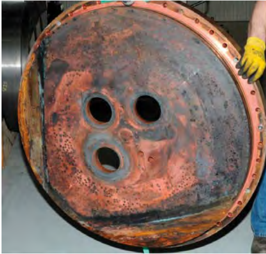
Corrosion products on the inside of the lid of the canister in deposition hole No 6. Corrosion have turned the copper surface black
