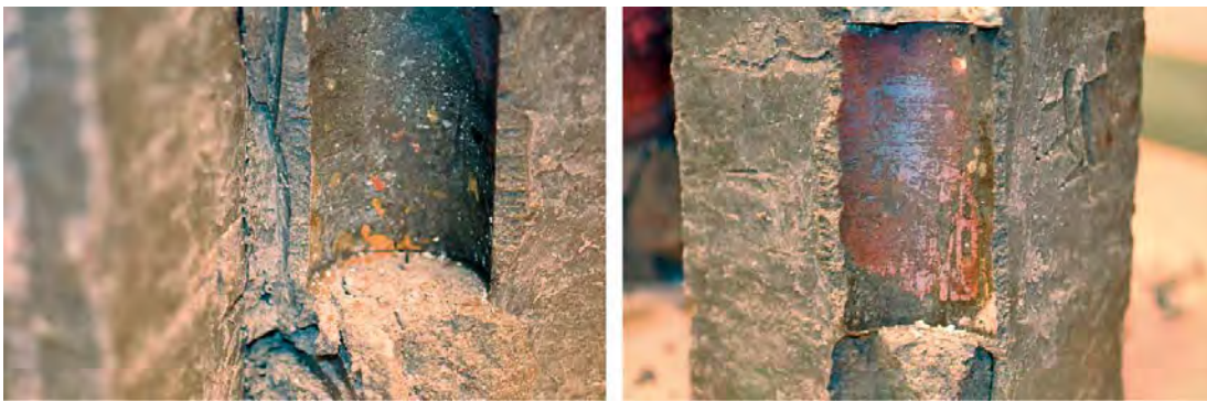
Figure 5-44. Corrosion products still remaining on adjacent bentonite after removal of the electrode. (Figure 3-1 in Rosborg 2013b.)
