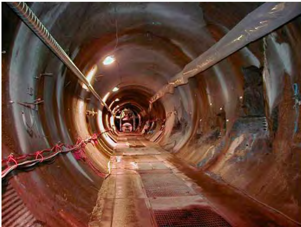
Figure 2-3. Prototype Repository tunnel with installed roadbed.
