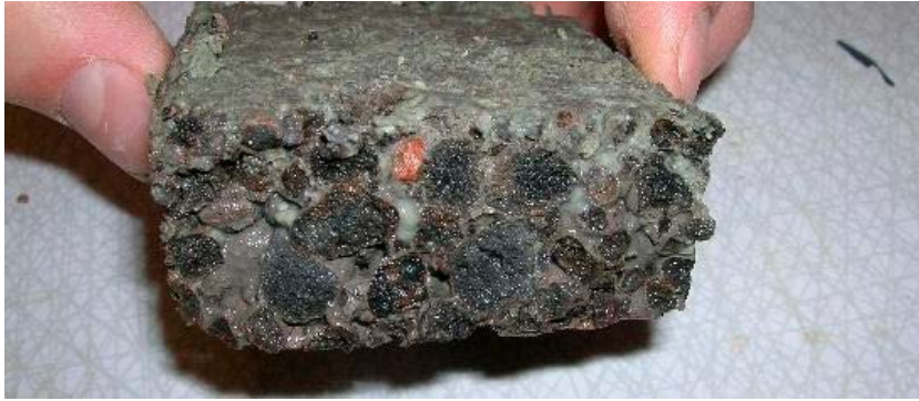
Figure 4-20. A cross section view of a Leca beam split in two. Backfill bentonite has intruded about half way through the 30 mm thick beam.
