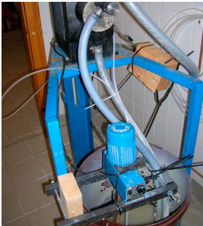
Figure 3-19. The bentonite-water slurry under constant agitation and the pump.
