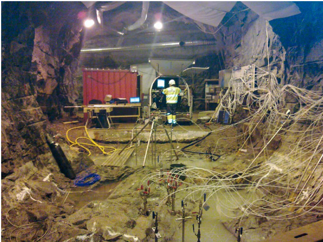
Figure 5-1. The location of the measured boreholes and the measurement trailer in the Äspö TASEO-tunnel.
