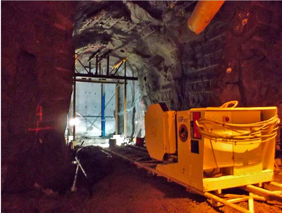
Figure 3-7. The wire saw machine mounted on rail.
