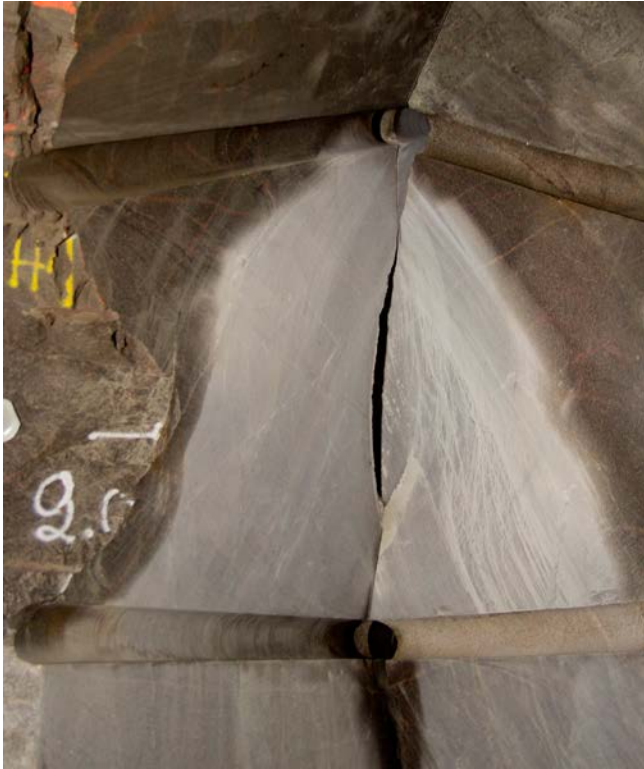
Figure 4-2. Detail photo of the left side crest of the excavated slot where a cavity occurred.
