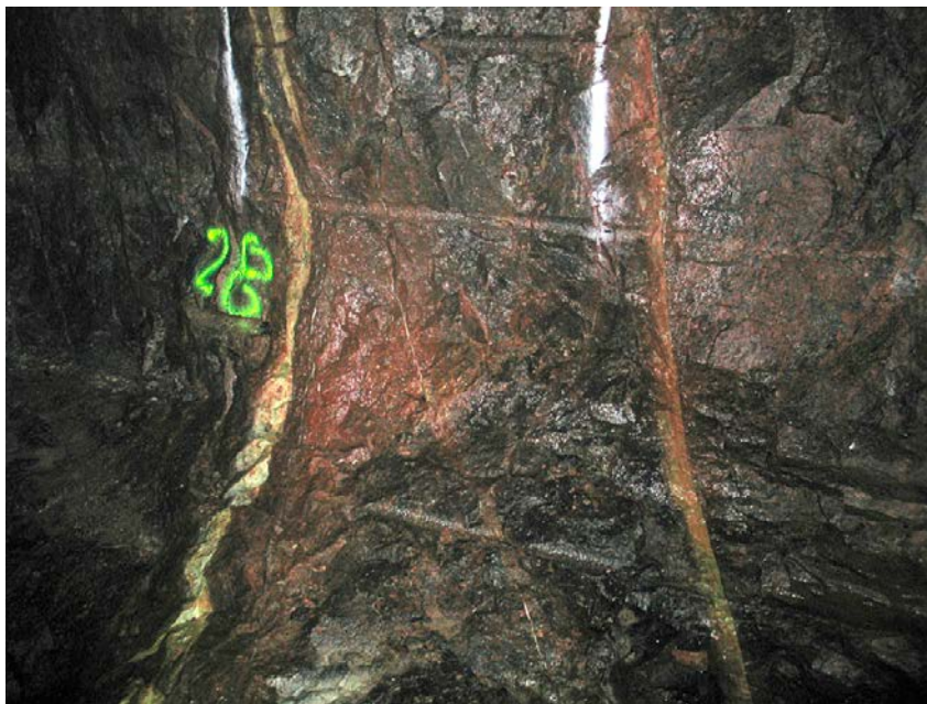
Figure 6-3. The deformation zone in TAS04. Photograph taken towards the left wall between approximately 28 and 29 m, showing the two cataclastic bands that define the zone.
