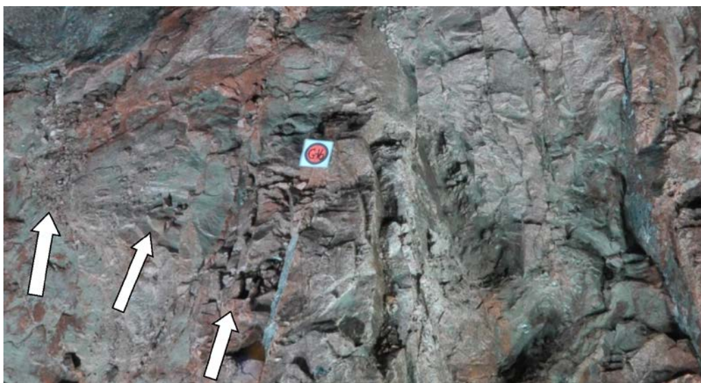
Figure 6-9. Enlargement from an RoCS-mapping photograph from the floor of TAS04 at approximately 19 m showing the fractured fine-to-medium-grained granite with the broken-up smaller pieces (some are indicated by the white arrows). The red circle is the coordinate point G16, measured with total station as an orientation for the 3D model (coordinates in ÄSPÖ96: X: 2429,588, Y: 7351,559, Z: -409,107).
