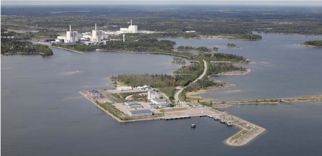
Figure 1-2. The surface part of the SFR facility in the harbour in Forsmark with the Forsmark nuclear power plant in the background.
