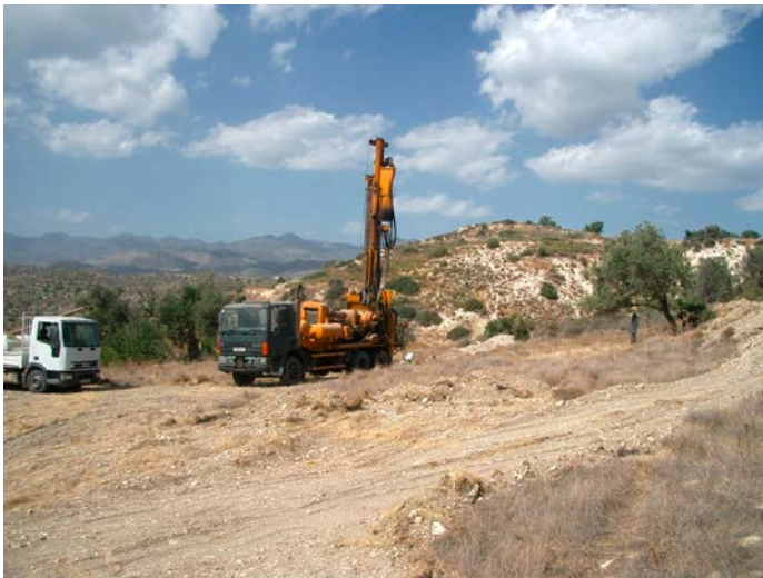
Figure 2-15. Drilling through the bentonite at Parsata, Cyprus. Samples are recovered throughout the bentonite column (up to 40 m thick here) and at the base of the column, overlying the pillow lavas which are the source of the alkali groundwaters.
