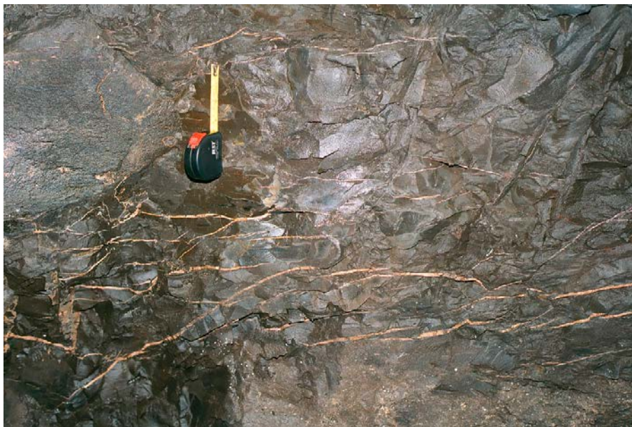
Figure 2-7. Example of sub-bedding parallel fractures and joints (here sealed by secondary tobermorite) in the clay biomicrite host rock at Maqarin (Pitty and Alexander 2011).
