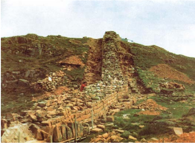
Figure 2-30. Section of Hadrian's Wall, northern England. The large stone blocks were held together with mortar (from Miller et al. 2000).
