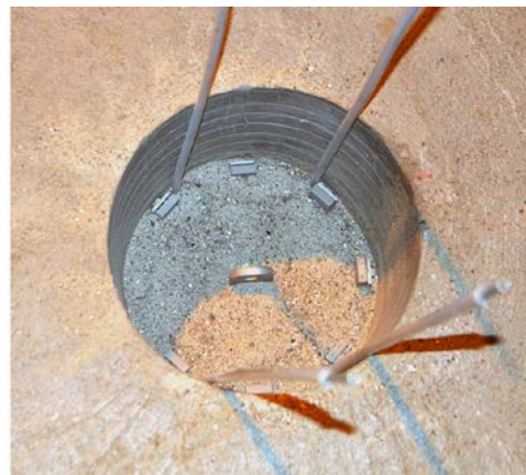
Figure 6-10. Filling the slit between the bentonite package and the rock wall as well as some of the volume on top of the bentonite package with sand.
