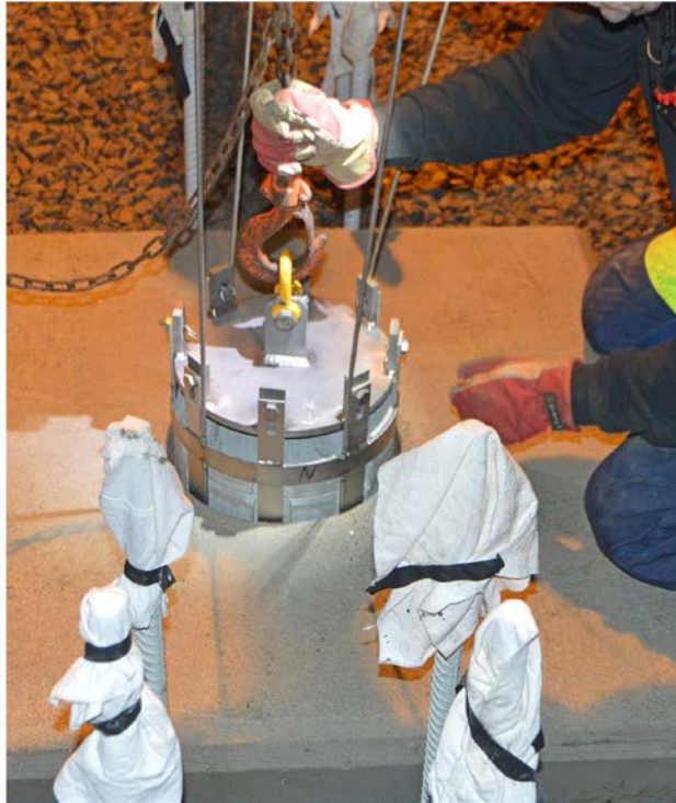
Figure 6-9. Lowering the bentonite package into the deposition hole. Please note the marking “N” on the titanium cage facing towards the end of the niche.
