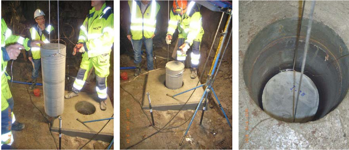
Figure 6-2. Installation of one of the concrete cylinders in the deposition hole.
