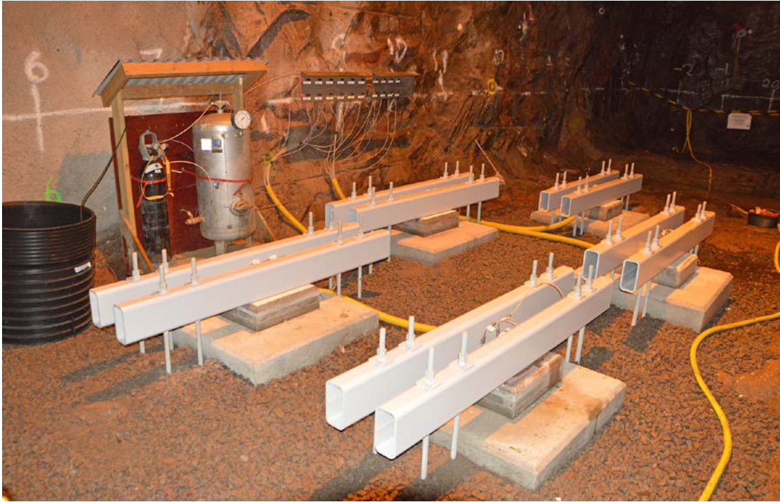
Figure 6-11. Installation completed and system for artificial saturation of the experiments connected.
