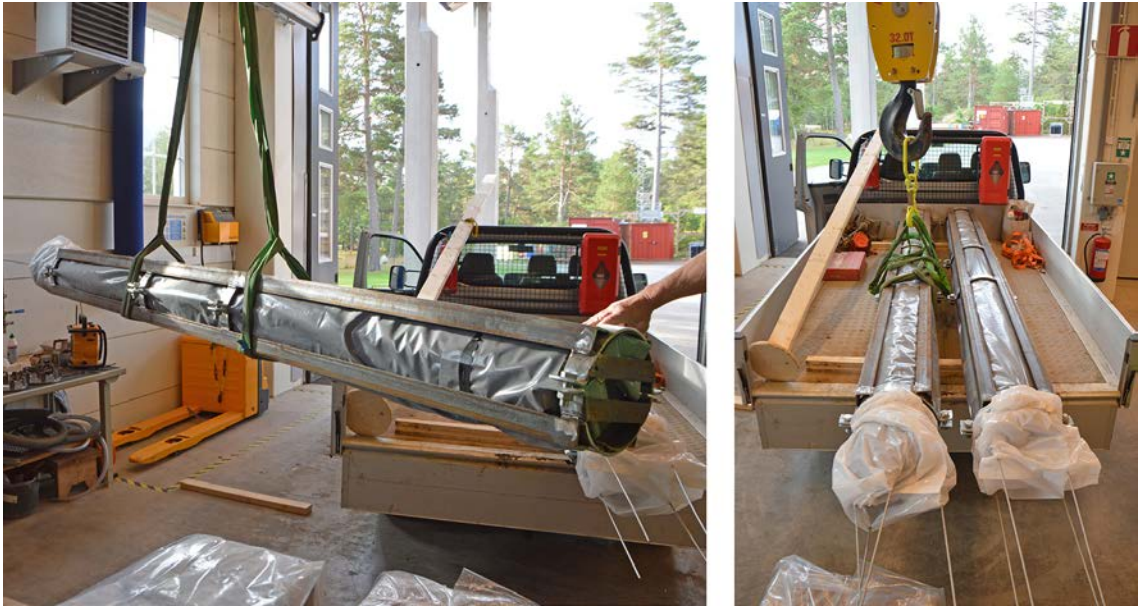
Figure 6-7. Loading the bentonite package onto the truck for further transport to TAS06.
