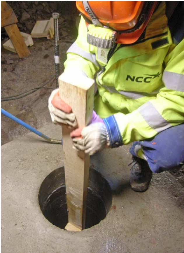
Figure 6-1. Levelling the bottom and measuring the depth of the deposition hole.
