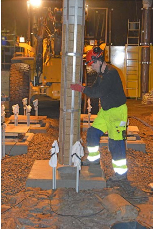
Figure 6-9. Lowering the bentonite package into the deposition hole. Please note the marking “N” on the titanium cage facing towards the end of the niche.
