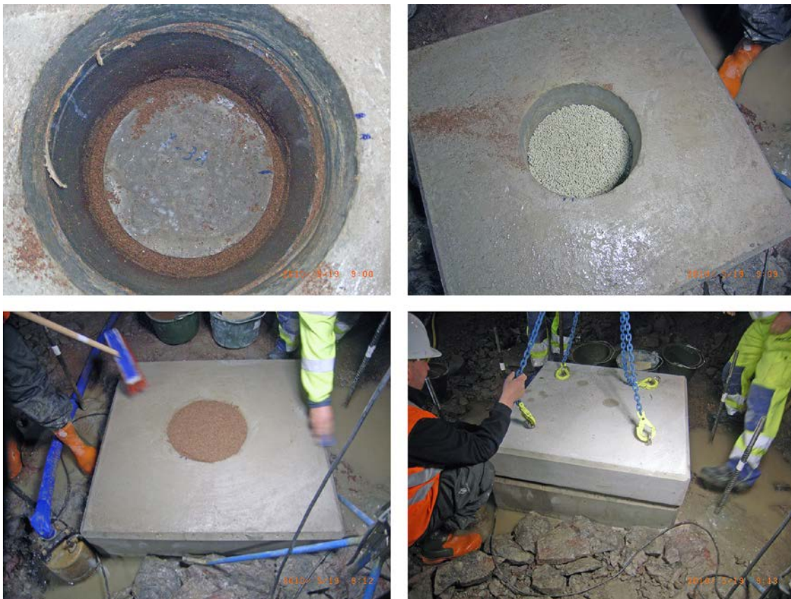
Figure 6-3. Sealing and closure of the field scale concrete experiments.
