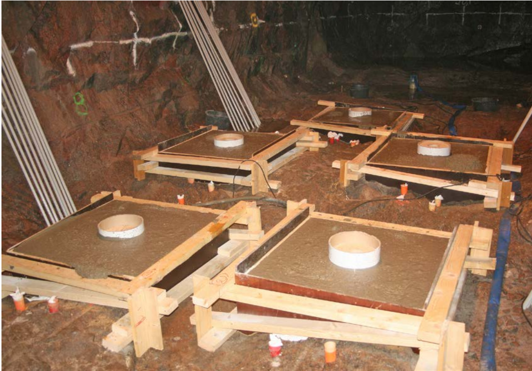
Figure 3-10. Casting of the bases in TAS06.
