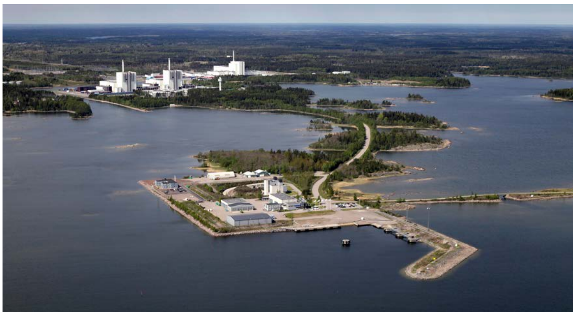
Figure 1-2. The surface facilities of SFR 1 in the Forsmark harbour.
