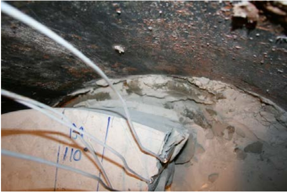
Figure 4-10. Bentonite with high water content in the gap between the block and the test cylinder.
