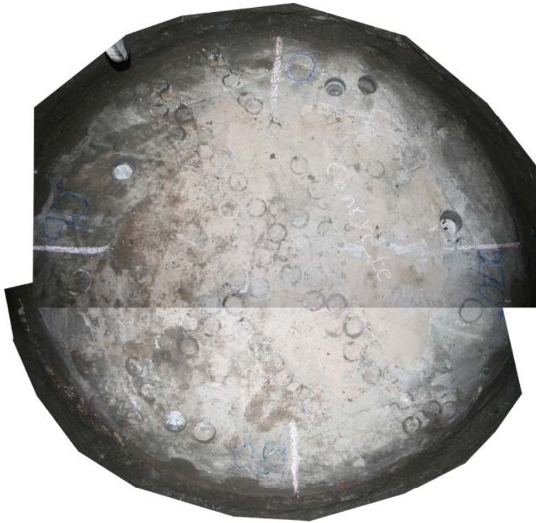
Figure 2-43. Concrete bottom plate.
