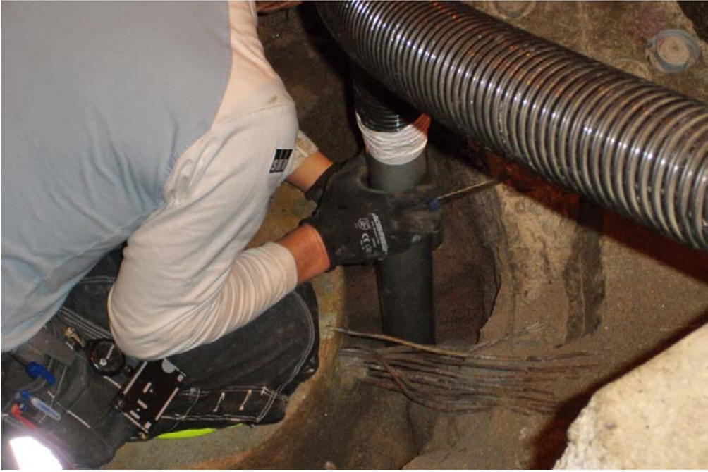
Figure 2-12. Sand removal with industrial vacuum cleaner.
