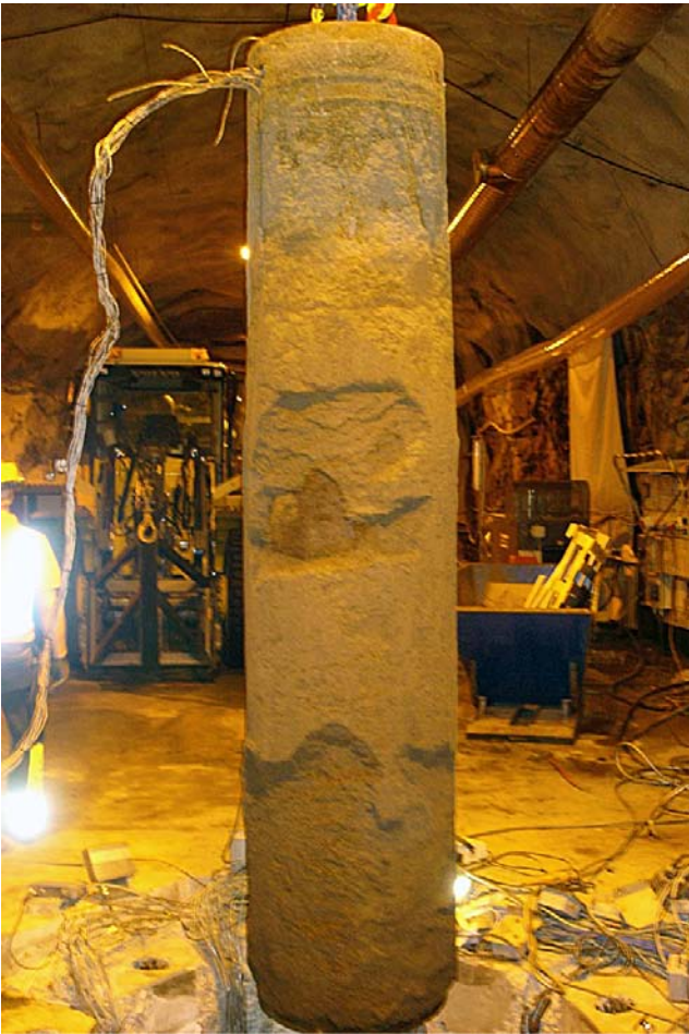
Figure 2-13. Lifting of Heater II.
