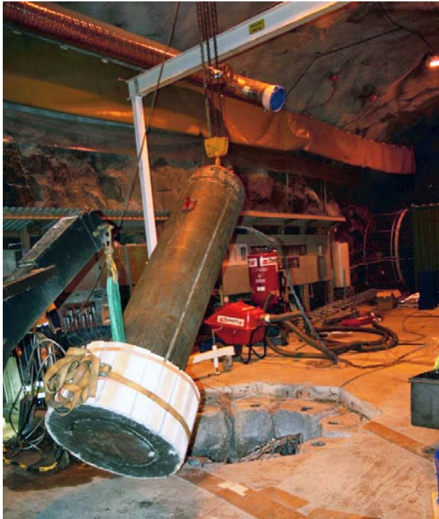
Figure 2-35. Lifting of Heater I.
