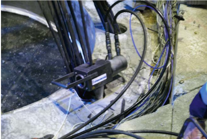
Figure 2-2. Cutting of anchor cables.
