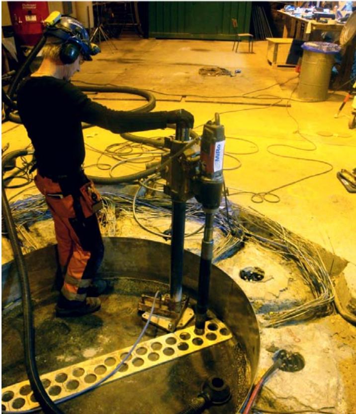
Figure 1-2. Coring machine used for sampling and partitioning of bentonite blocks.
