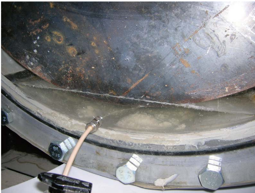
Figure 9-24. View on conclusion of the erosion measurement. (The amount of bentonite on the tunnel floor had increased so much that the drainage was prevented and the water level rose above the supercontainer base).
