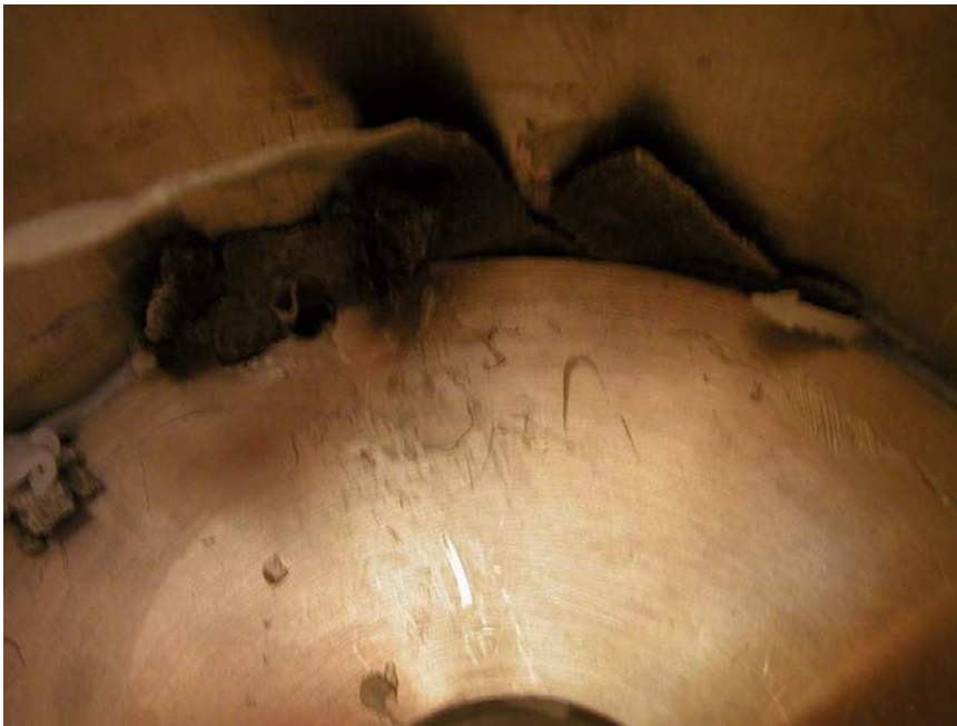
Figure B8-3. Picture showing the fixing ring. Bentonite was squeezed out between the ring and the steel tube.
