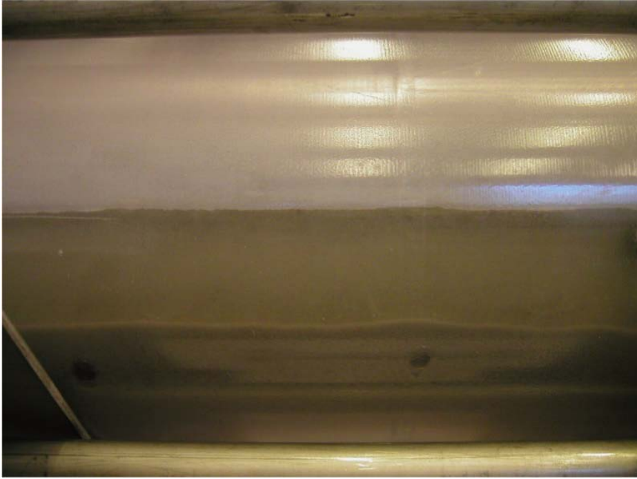
Figure 7-29. Photo taken during the pre-wetting of the outer slot. Water has filled half way up and bentonite has discharged from the blocks and settled to the bottom.
