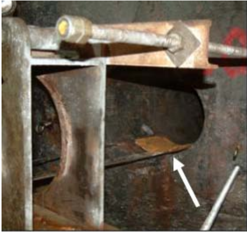
Figure 5-3. Insertion of tool for core breakage.
