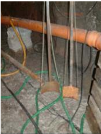
Figure 5-2. Tools for core breakage.
