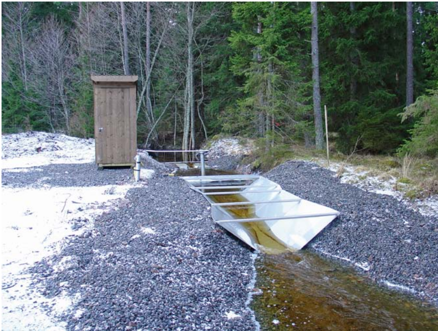
Figure 3-1. Discharge station PFM002667 with the large flume in the foreground, the small flume upstream in the background, and the service module with the LPG burner used for de-icing to the left. The tube in the middle of the brook, between the flumes, is screened and contains the devices for measurement of electrical conductivity and temperature.
