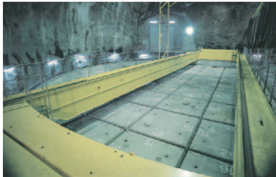
View over top of silo
