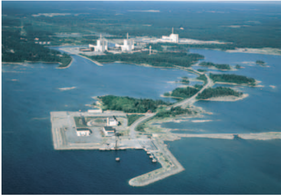
View of the surface part of SFR (the Forsmark NPP can be seen in the background)
