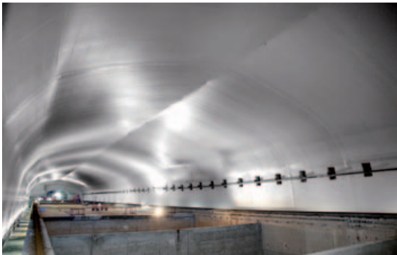
Rock vault for intermediate-level waste
