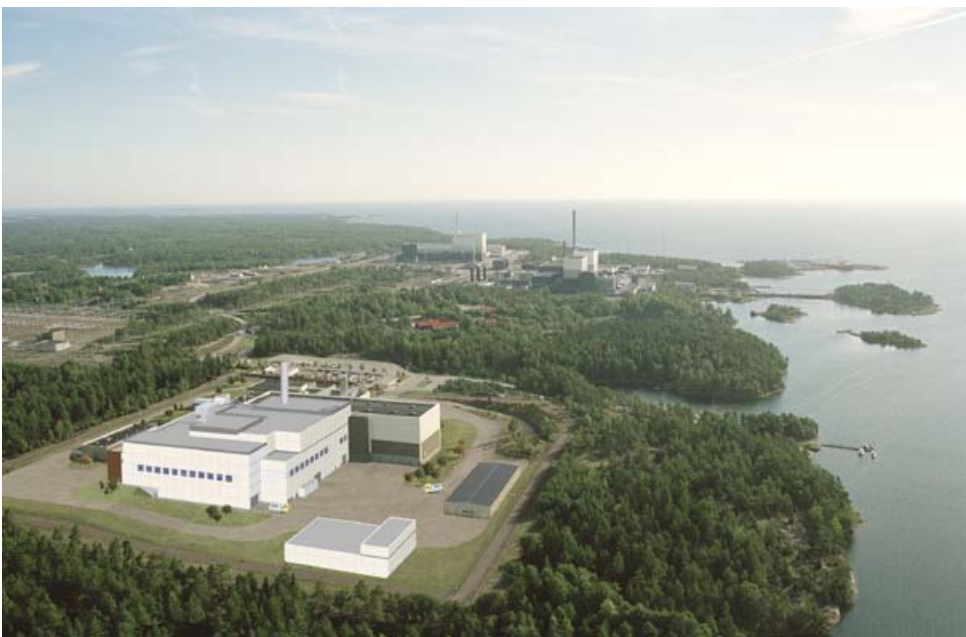
Figure 2-8. Encapsulation plant for spent nuclear fuel integrated with Clab.
