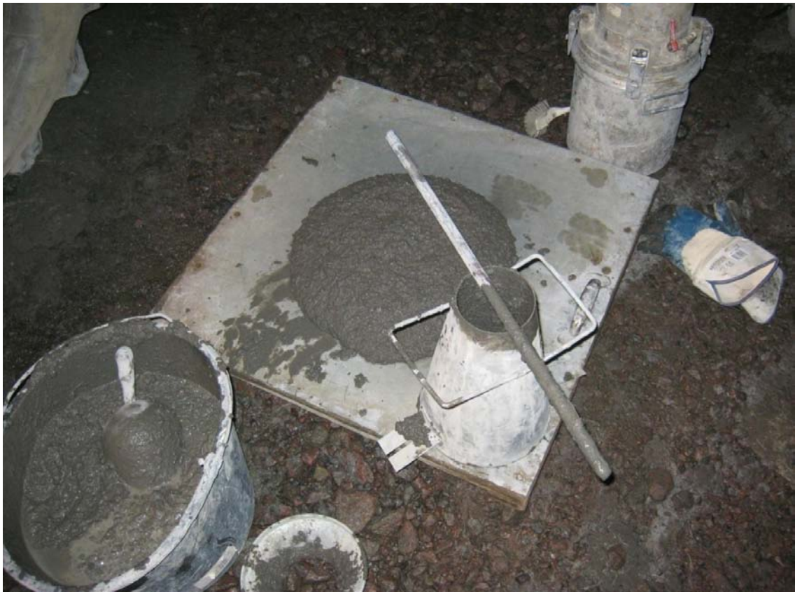
Figure 4-2. The workability of each batch was slump tested.
