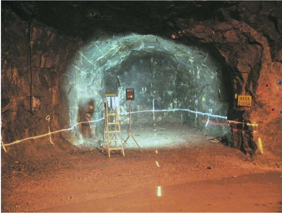
Figure 3-3. Niche NASA0408A. This photo was taken by Magnus Kronberg SKB as part of the preparation for the field test.
