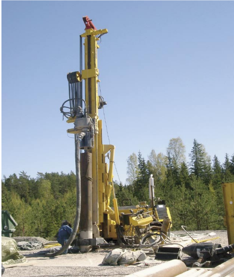
Figure 3-2. The Puntel drilling machine engaged for drilling borehole HFM19.
