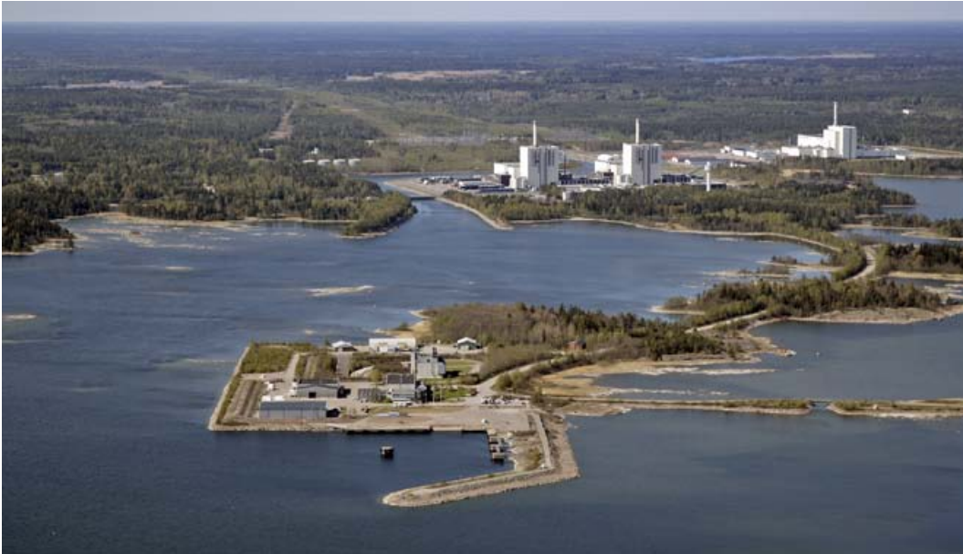
Figure 5-6. Aerial photo of Forsmark. Söderviken is located to the left of the nuclear power plant, with the cooling water channel visible between them. In the foreground is the SFR facility.
