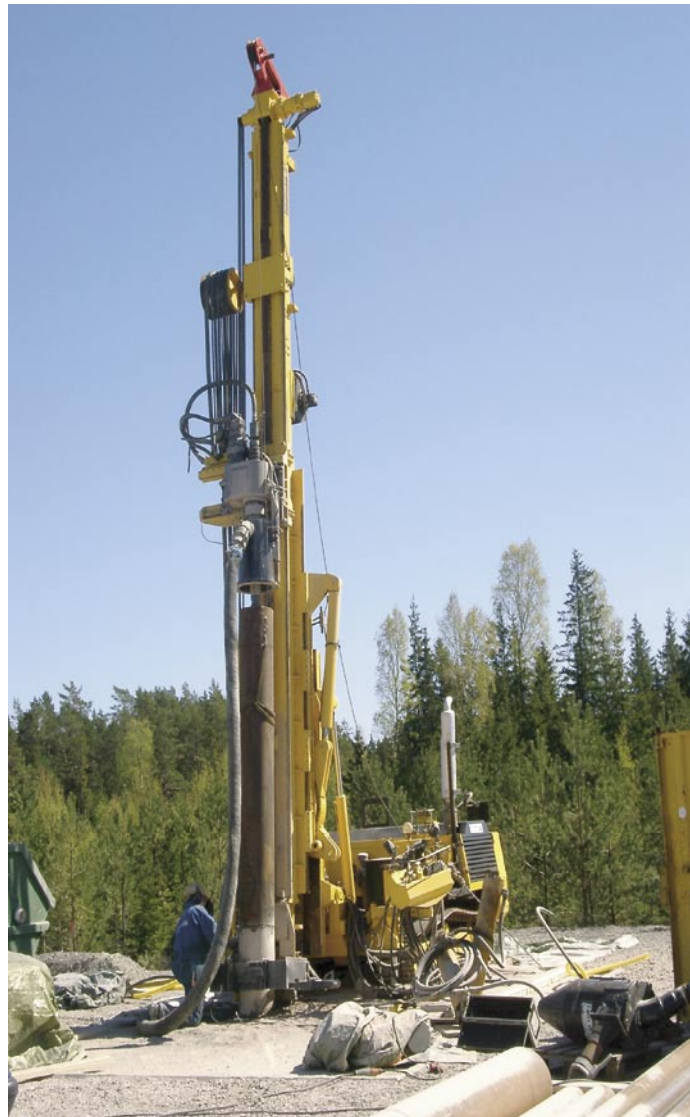
Figure 3-1. The Puntel drilling machine in operation.
