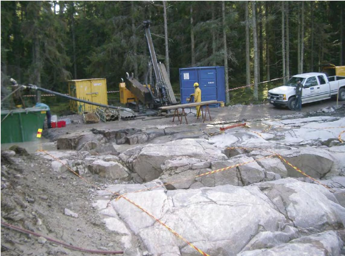
**Figure 3-1.** The Nemek 407 percussion drilling machine employed for drilling wells in rock and soil at drilling site DS5. Water and drilling debris is discharged to the container to the left. The fractured out-cropping bedrock, after un-covering of the till layer, is shown in the foreground.
