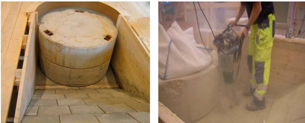
Figure 5-16. Backfilling of bevel at Äspö HRL
