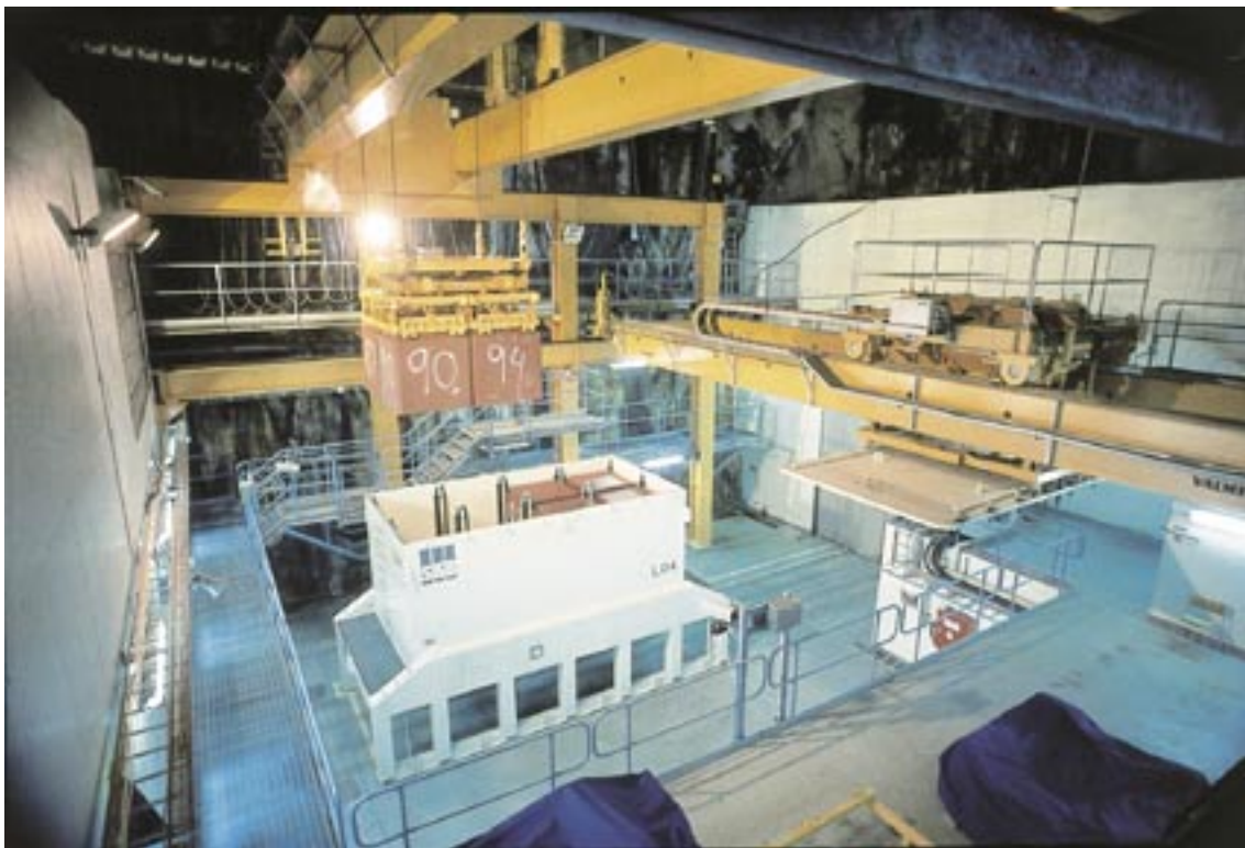
Figure 3-4. Photo from unloading the transport container at SFR.
