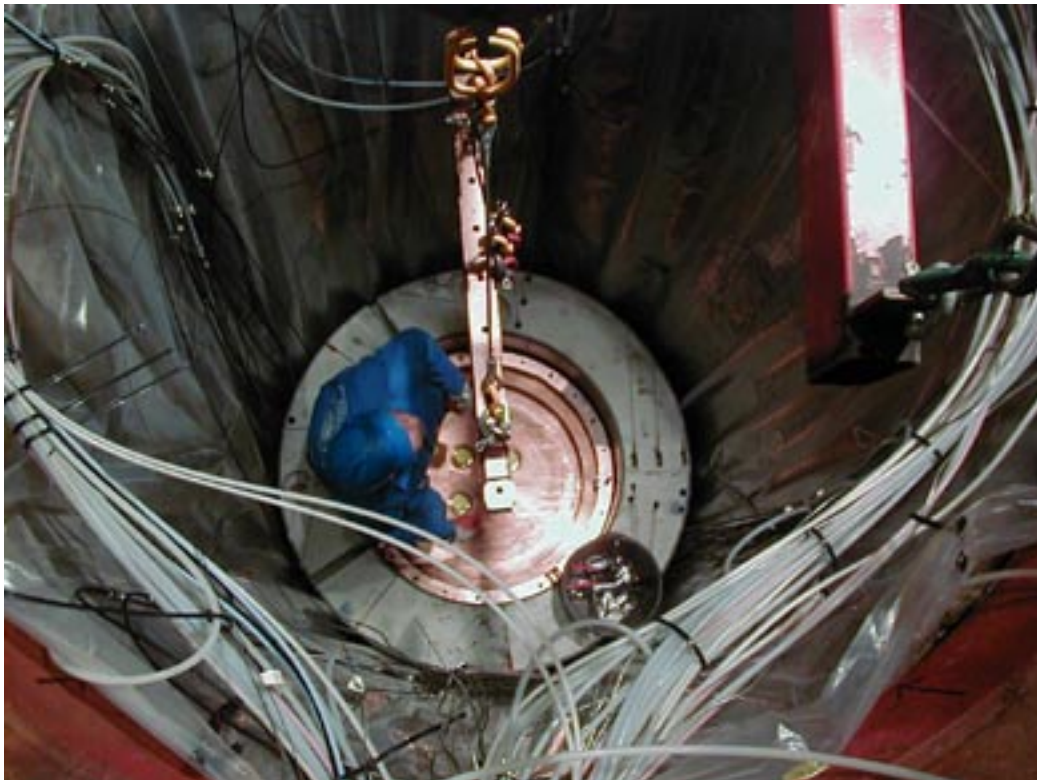
Figure 3-9. Photo showing installation of displacement sensors on top of the mock-up canister.
