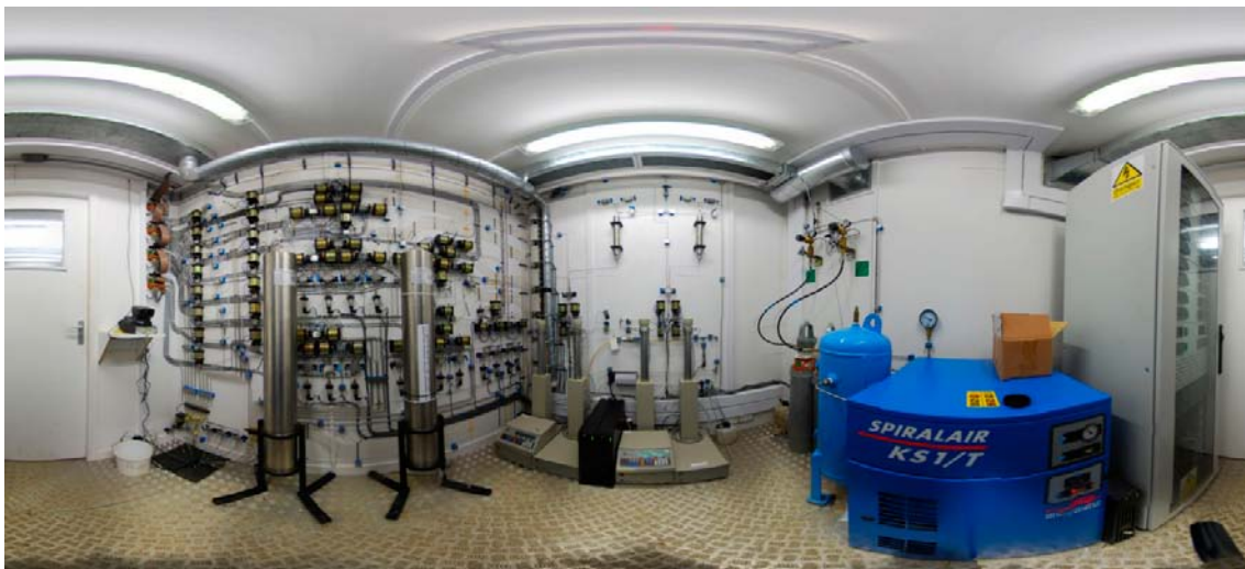
Figure 4-21. Panorama of the laboratory area for the large-scale gas injection test at the –420 m level at Äspö HRL.
