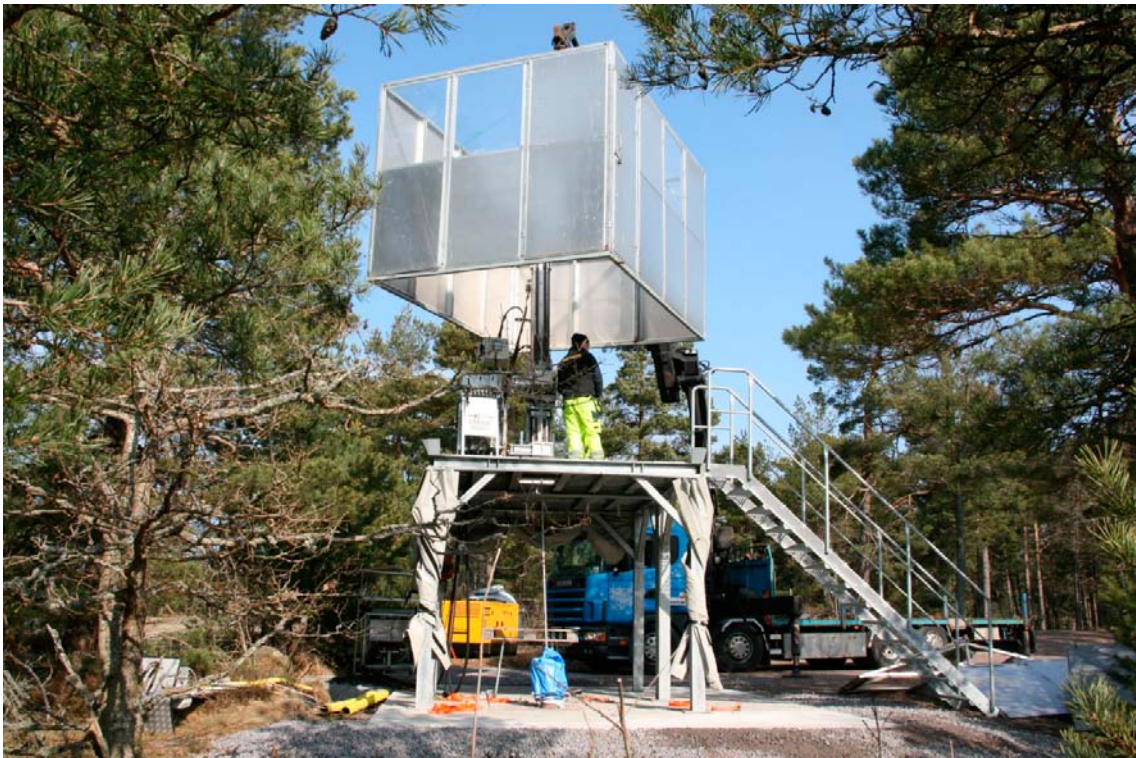
Figure 2-3. Site mobilisation for retrieval of monitoring equipment from borehole KAS09.
