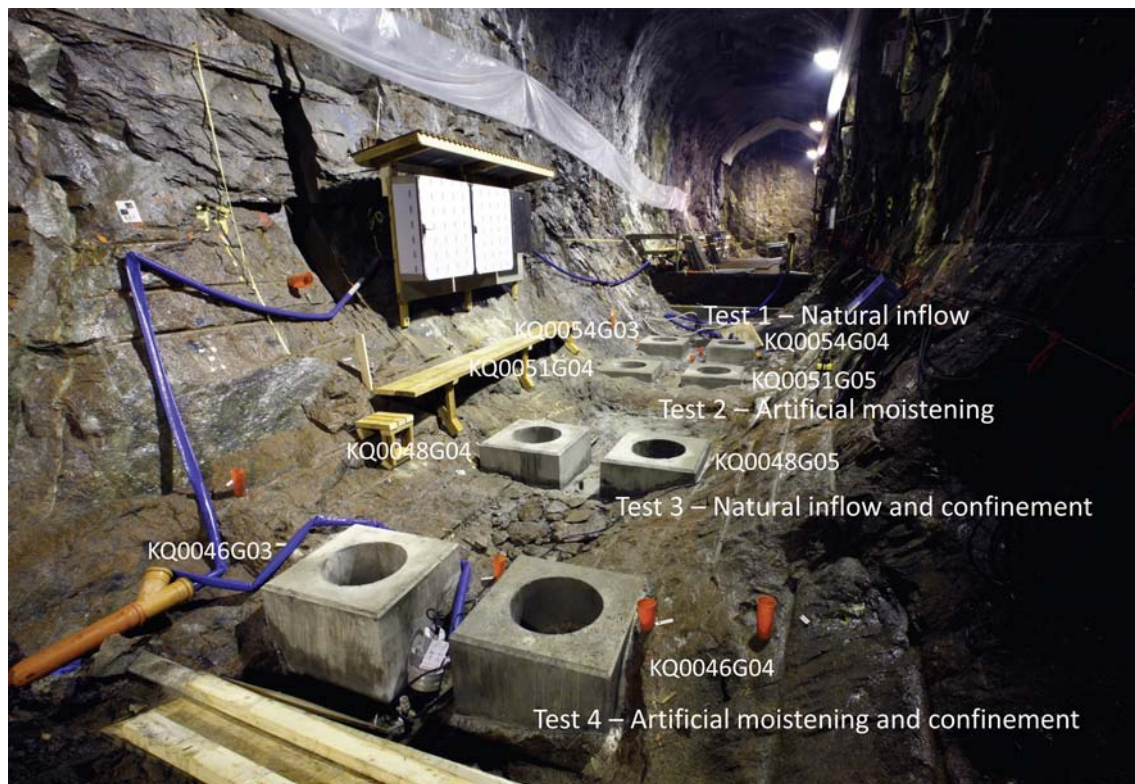
Figure 2-5. The test site of Caps in the Tasq-tunnel at Äspö HRL. The photograph was taken before all of the instrumentation holes had been drilled. The test sequence of the field experiment as well as labels of the heating holes, are indicated in the figure (Photo C-R Lindqvist).
