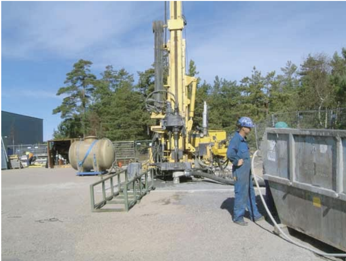
Figure 2-1. The percussion drill rig.
