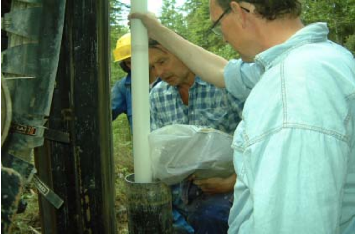
Figure 4-1. Installation of the HDPE well screen, riser pipes, sand filter and bentonite sealings in a groundwater monitoring well inside a temporary steel casing. The snapshot illustrates filling with bentonite pellets. Photo Göran Nilsson.
