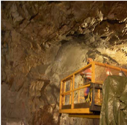
Field test with low-pH shotcrete at Äspö HRL executed within the EC project ESDRED in 2006.
