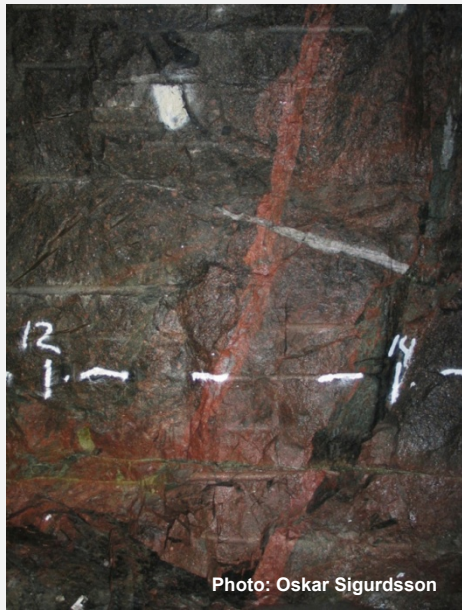
The TASS-tunnel, left wall, section 12-14 m. In the lower part a sub-horizontal, epidote healed fracture displacing a pegmatite dyke and in the middle a quartz lens cross-cutting the same dyke.
