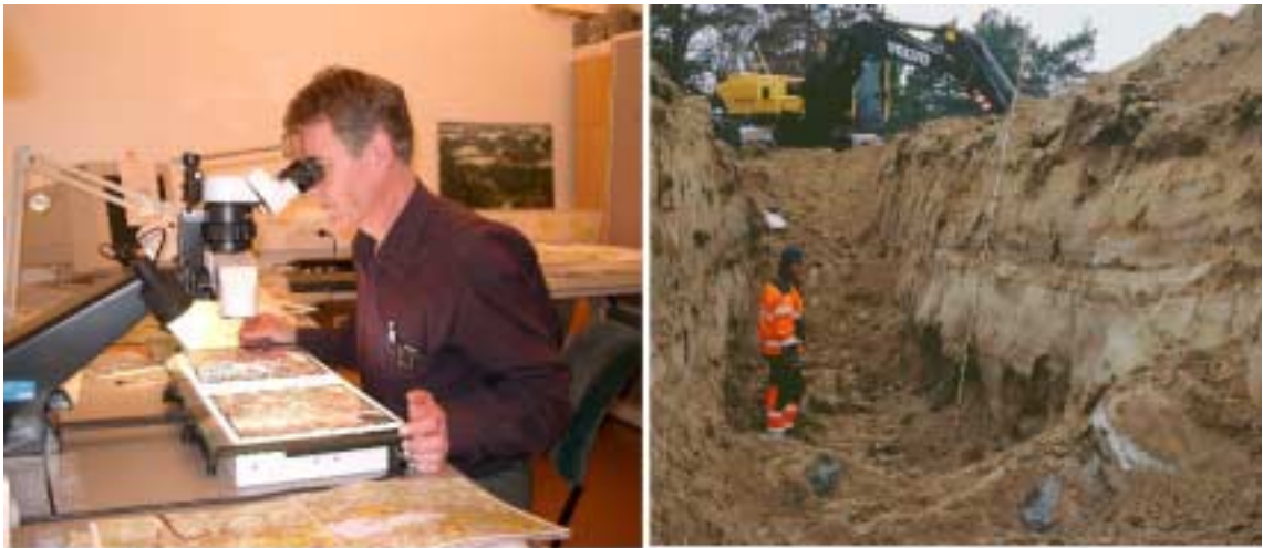
Figures 3-1 and 3-2. Air-photo interpretation and stratigraphical investigations in machine-cut trenches are the most important steps in the investigation.
