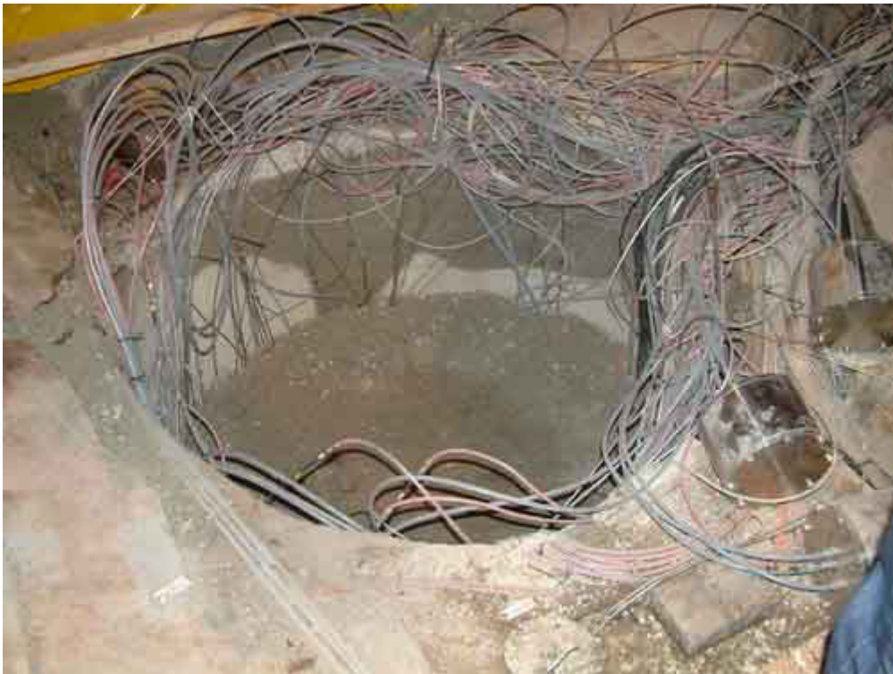
Figure 2-1 Deposition hole 5 in Section II of the Prototype Repository. The picture shows the top of the upper most bentonite block and cables which connect instruments in the bentonite block with the measuring units located in an adjacent tunnel.
