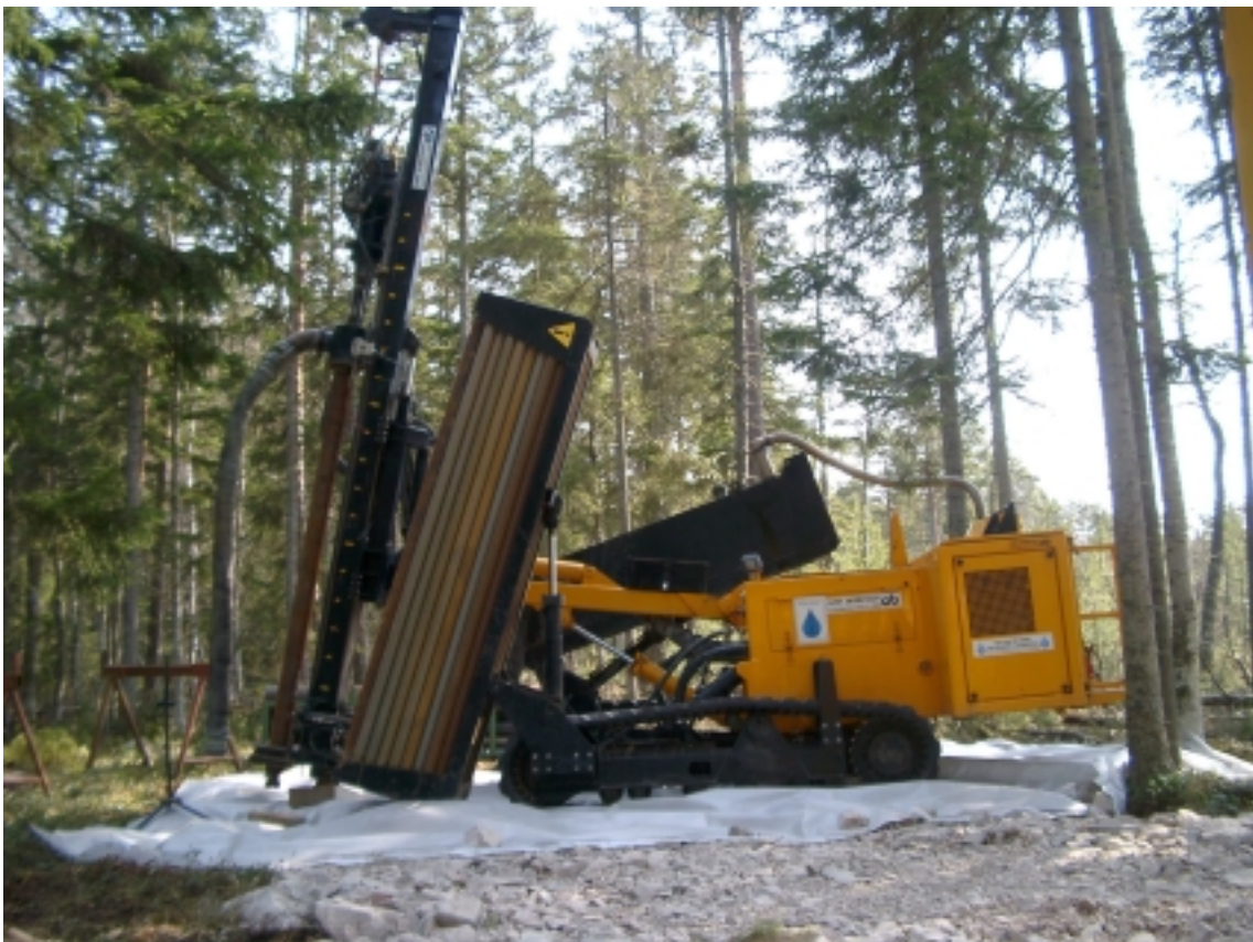
Figure 3-1. The Nemek 407 percussion drill machine engaged for drilling the monitoring wells in unconsolidated soil layers. Note the fluidproof cover beneath the drill rig used for protection of the ground in case of unintentional oil spillage. Photo Alf Sevastik.
