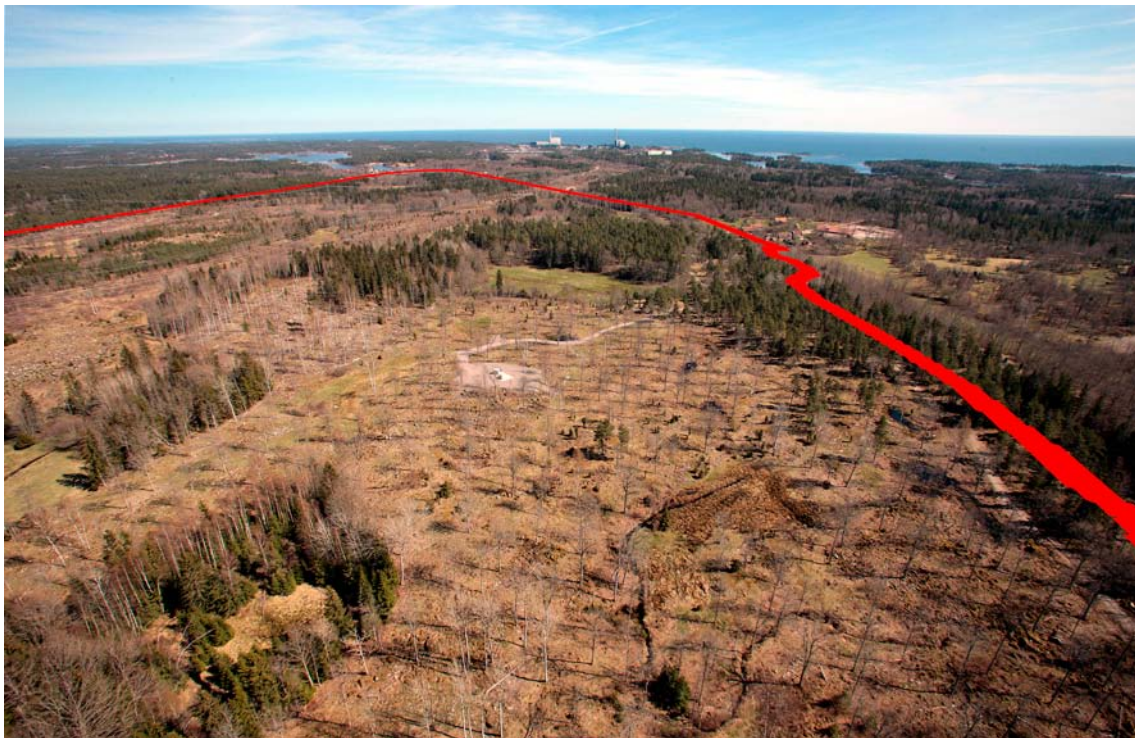
Figure 1-5. Air photographs showing the flat topography, low gradient near shore situation in the Laxemar-Simpevarp area with shallow bays, a) view from the southeast, Clab facility in the foreground, b) view from the west, drill site KLX05/KLX12A in the centre of the photograph. Both photographs show the outline of the focused area in Laxemar in red, cf. Figure 1-6.
