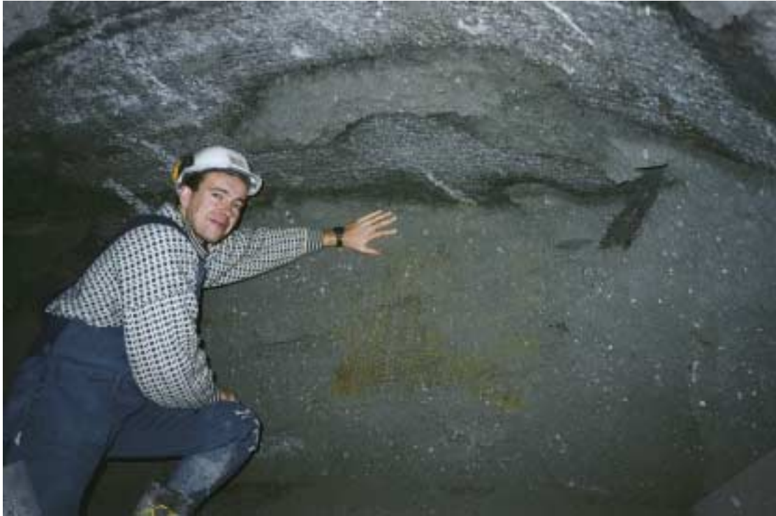
Figure 9-10. Excavation of 10/90 backfill in backfilling experiment at Äspö. The backfill material adheres to the rock at wet spots.
