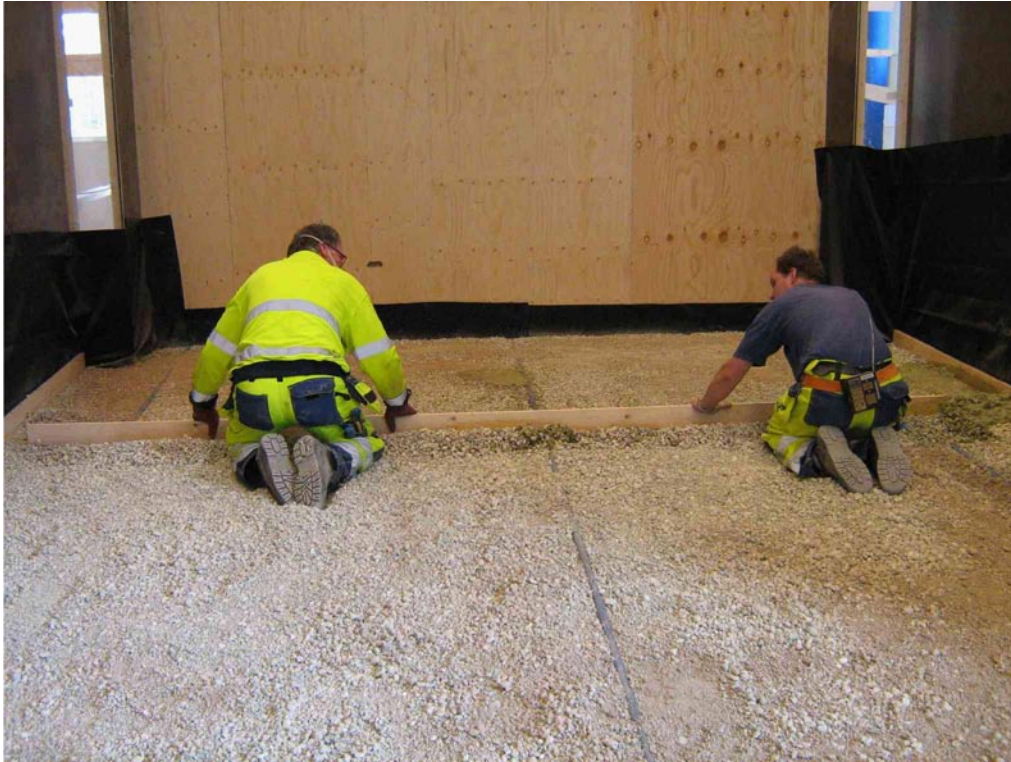
Figure 7-5. Preparation of the bottom bed using Minelco granules.
