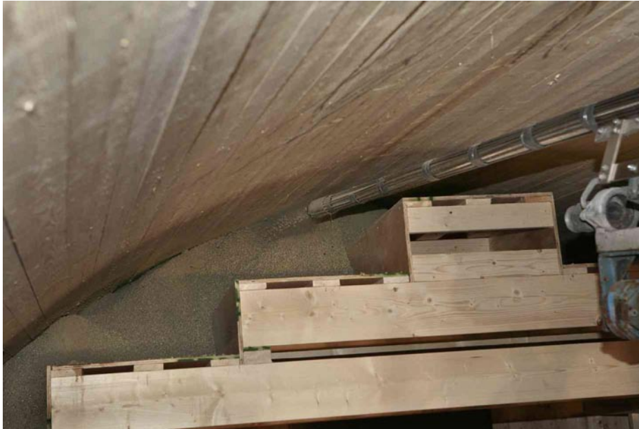
Figure 7-12. Pellet filling in the most narrow tunnel section.
