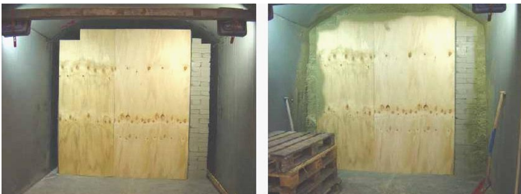
Figure 6-28. Tests where only a small volume of block materials installed. (Pellets installed into remaining volume and downstream face sealed through use of wet pellet materials.)
