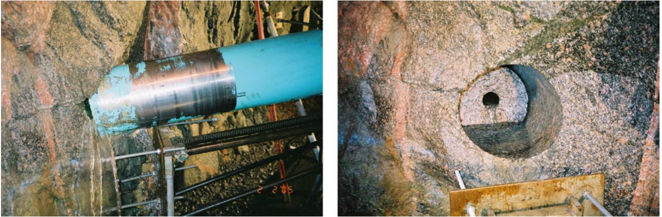
Figure 5-1. Preparation of boreholes for miniature canister experiments.
