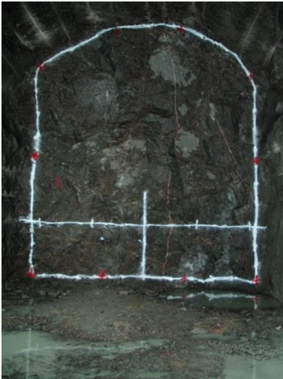
Figure 2-1. Tunnel front in the excavated Tass-tunnel.
