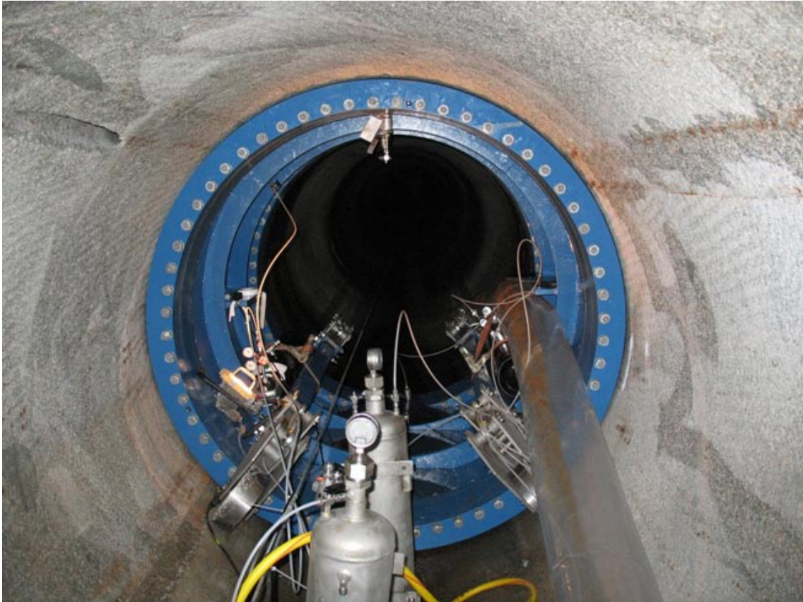
Figure 4-23. The MegaPacker used for grouting.
